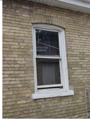
Image 4: Side elevation – east, showing existing window opening
