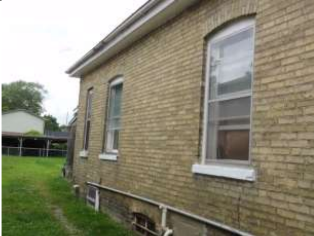
Image 3: Side elevation – west, showing existing window openings
