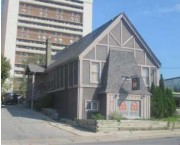
Image 5: 36 York Street, current (Stantec, Heritage Impact Statement )
