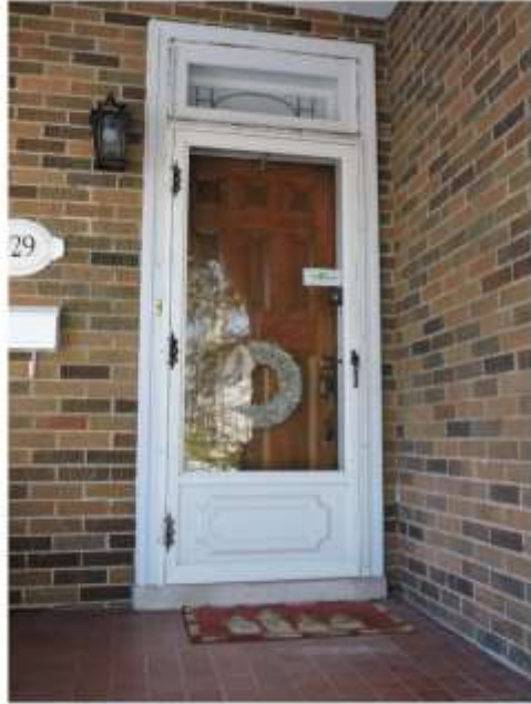
Figure 25: View of front doorway showing the original wooden door and rectangular stain glass transom (A. Barnes, 2017).
