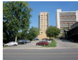
32 York Street Asphalt parking lot no structures
