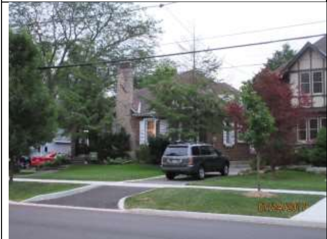
Image 3: View looking southeast of the property at 329 Victoria Street.
