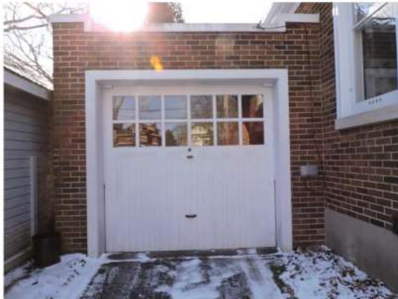
Figure 22: One storey brick garage with wooden door. The garage is attached directly to the western elevation (A. Barnes, 2017).
