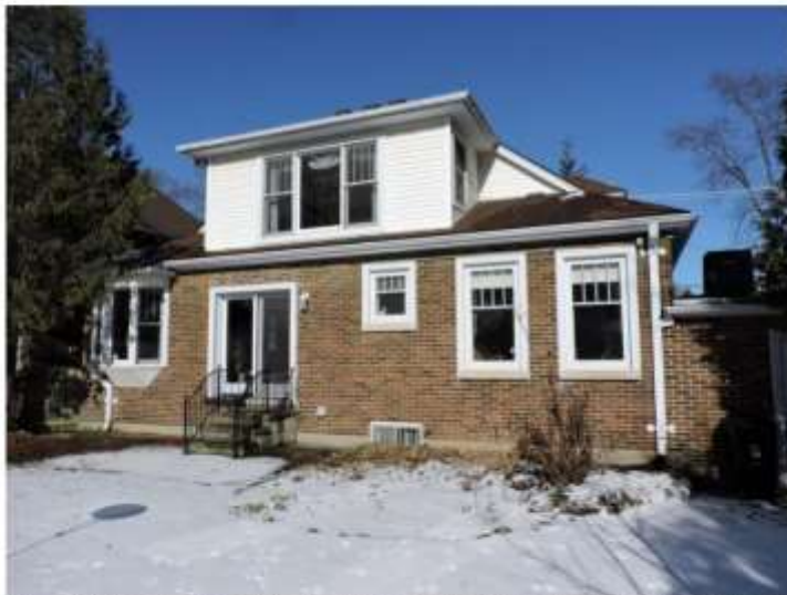
Figure 20: Rear of the property (south elevation). Note the upper level addition (A. Barnes, 2017).
