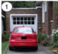
One and a half storey residential building with attached garage
