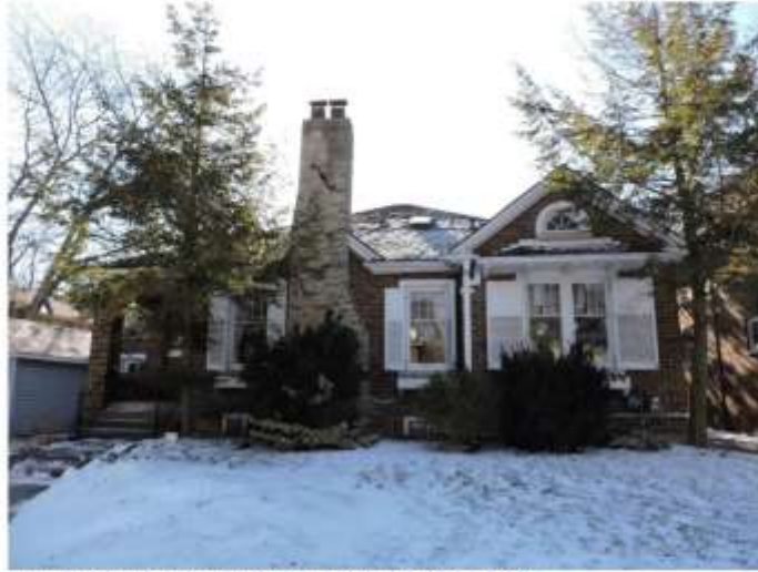
Figure 17: Front façade of 329 Victoria Street (A. Barnes, 2017).
