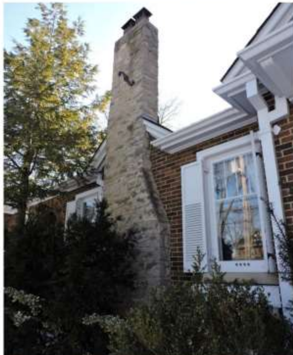
Figure 18: Detail of the stone chimney. Note the cut in the roofline (A. Barnes, 2017).
