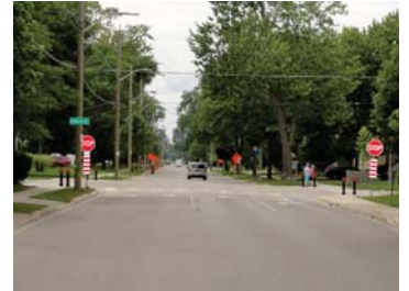
west view, towards Colborne and Grey Intersection
