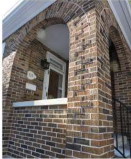
Figure 23: Western view of the open front porch showing the raised brick motif found along both arcade arches of the porch (A. Barnes, 2017).
