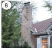
Large stone chimney
