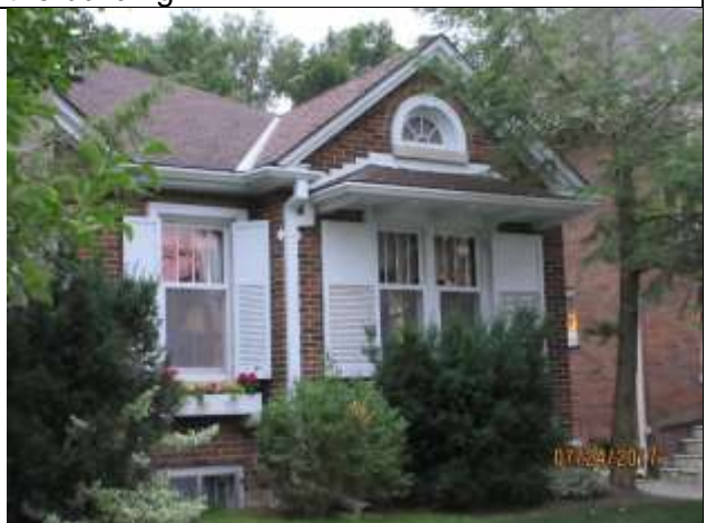
Image 6: Detail of the west end of the main façade showing the shutters, 4-over-1 wood windows, half round window, awning with wood soffit and modillions.
