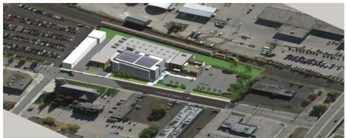
15-026 Start.ca | 639 York Street, London ON | Google Earth | April 2017 | A-18 | zedd ARCHITECTURE
