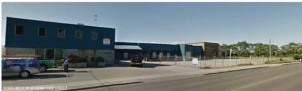
15-025 Start.ca | 639 York Street, London ON | Existing Site Imagery | April 2017 | A-03 | zedd ARCHITECTURE
