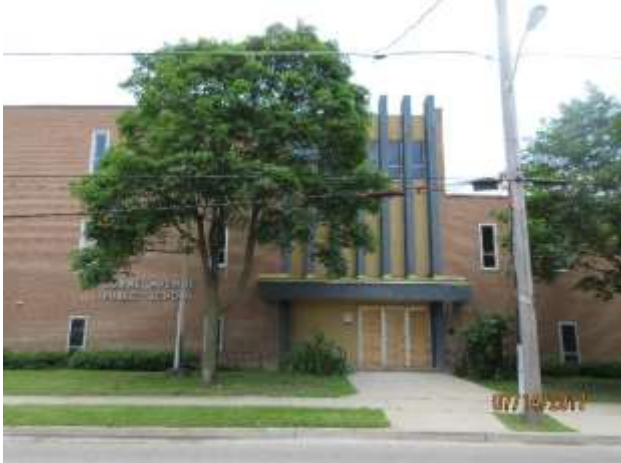
Image 18: Detail of the main entrance (north) to the Lorne Avenue Public School building.
