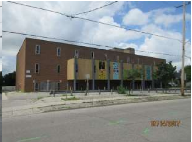
Image 13: East façade of Lorne Avenue Public School, see from English Street.
