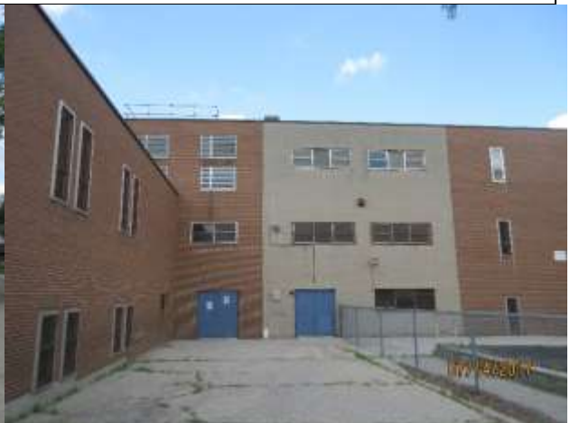
Image 15: South façade of Lorne Avenue Public School showing 1961 structure in contrasting cladding.
