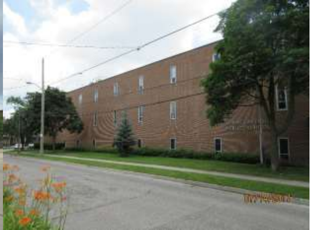
Image 17: North façade of the Lorne Avenue Public School building along Lorne Avenue.
