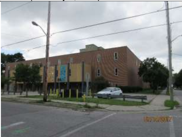
Image 12: View of Lorne Avenue Public School building from Lorne Avenue and English Street.
