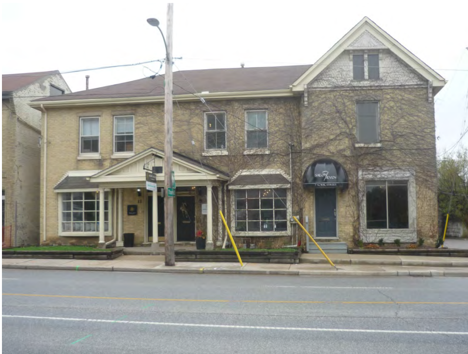
Plate 15: View of 7-11 York Street
