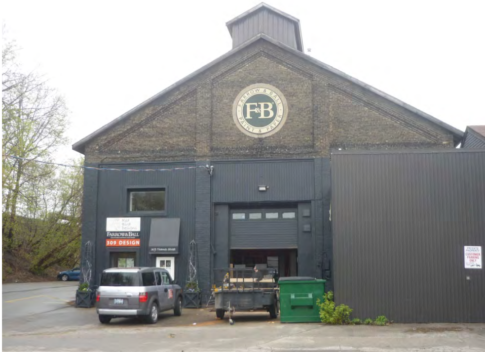
Plate 14: View of 309 Thames Street looking west from Thames Street
