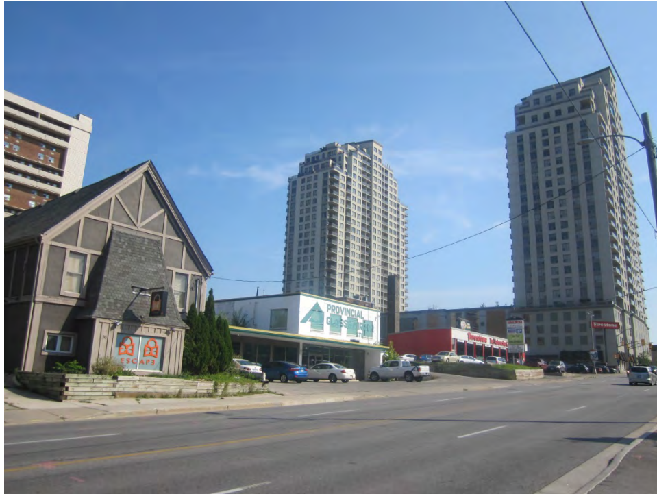
Plate 26: View looking northeast along York Street to Ridout Street
