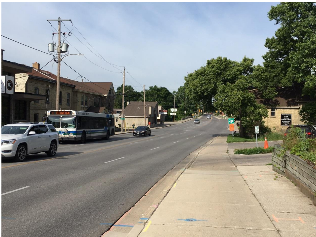
Image 4: York Street Streetscape, Northwest View taken from near 36 York Street, June 2017
