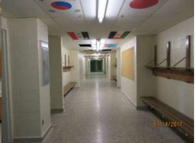
Image 21: Typical corridor of Lorne Avenue Public School (Corridor 3B).
