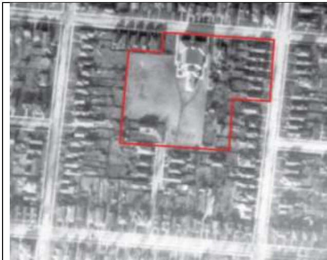
Image 1: Aerial photograph of the Lorne Avenue Public School showing property with original school building (1922, R290).
