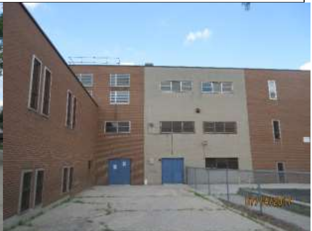
Image 15: South façade of Lorne Avenue Public School showing 1961 structure in contrasting cladding.
