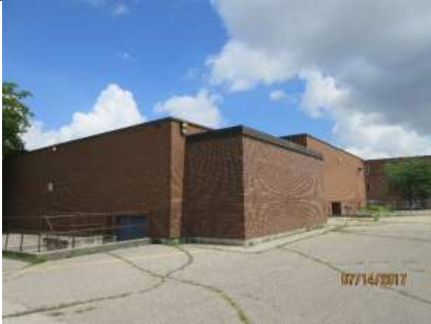
Image 16: Southwest wing of the Lorne Avenue Public School building, comprising the gym.
