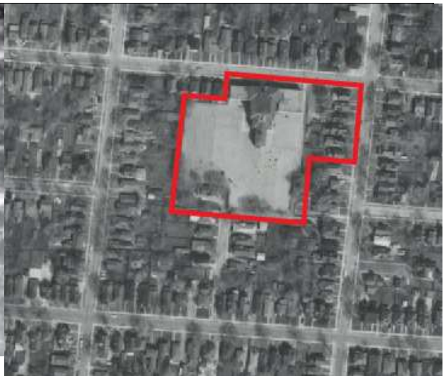
Image 2: Aerial photograph of the Lorne Avenue Public School property showing the 1956 and 1961 additions to the original school building (1965, Line 5, Image 209).
