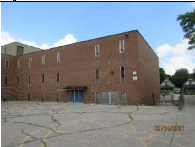
Image 14: Southeast wing of the Lorne Avenue Public School building seen from the playground.
