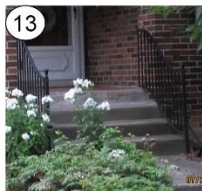
13 Wrought iron railing and terra cotta tile at entrance-way
