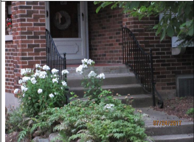
Image 5: Detail of the front stoop, with wrought iron railing, terra cotta tile, and brick pier.
