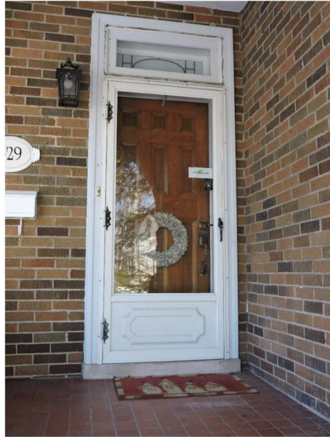
Figure 25: View of front doorway showing the original wooden door and rectangular stain glass transom (A. Barnes, 2017).
