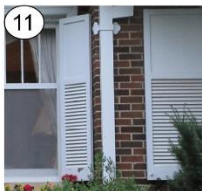
11 Original wood shutters
