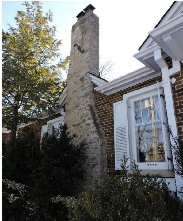
Figure 18: Detail of the stone chimney. Note the cut in the roofline (A. Barnes, 2017).
