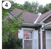
4 Hipped roof, overhanging eaves, moulded soffit, simple frieze
