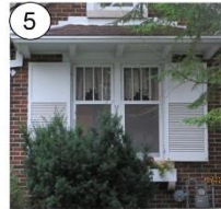
5 Small hipped roof over the double window with soffit and modillions
