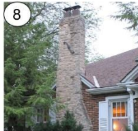
8 Large stone chimney
