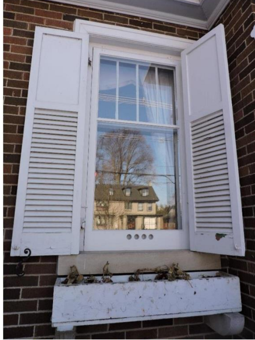
Figure 19: Details of the double hung, 4 over 1, wooden windows and wooden shutters. The storm windows are newer (A. Barnes, 2017).
