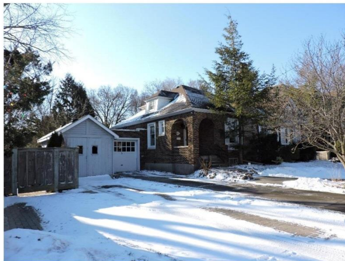
Figure 16: Western elevation of the property, showing the proximity of the driveway and shed of the adjacent property (white building on the left) (A. Barnes, 2017).
