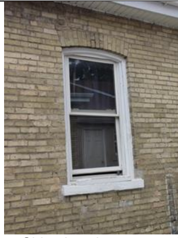
Image 4: Side elevation – east, showing existing window opening
