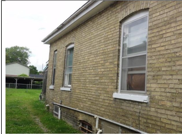
Image 3: Side elevation – west, showing existing window openings
