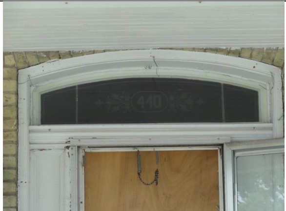
Image 6: Transom with etched coloured glass
