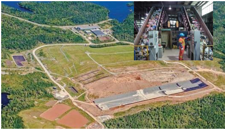
Otter Lake Facility Halifax, Nova Scotia – 3 facilities at 1 location
