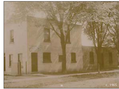
This is the former Kent Brewery, on Ann Street, established in 1859.
