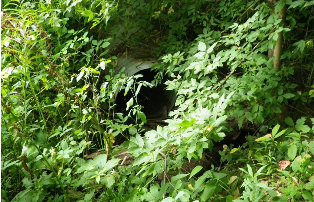
Photo 15 - Reach DCT-3 . Southdale Road West crossing at downstream limit.
