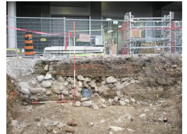
An example of a stone and brick foundation
