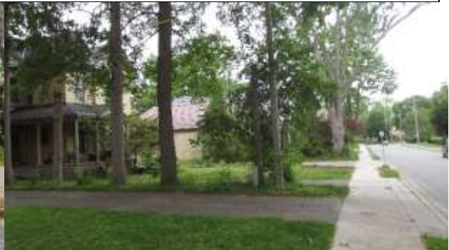
Image 4: View looking north showing the setback of the buildings along the west side of Marley Place (June 13, 2017).
