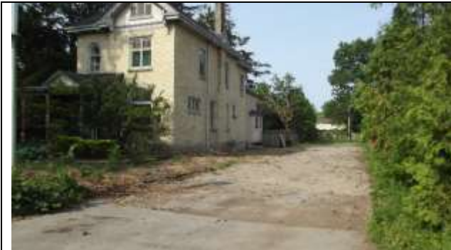
Image 1: The vacant property at 21 Marley Place, showing the building at 23 Marley Place to the south (left) (June 13, 2017).
