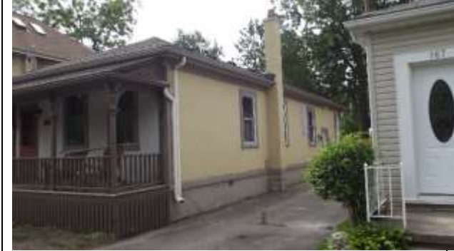
Image 7: West façade of the building at 169 Bruce Street showing the chimney (2017-06-13).
