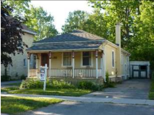
Image 1: Building at 169 Bruce Street (2016-06-14).
