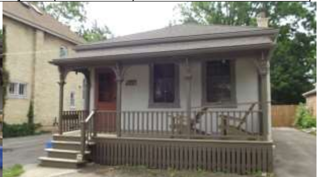
Image 6: Recent image of the building at 169 Bruce Street (2017-06-13).
