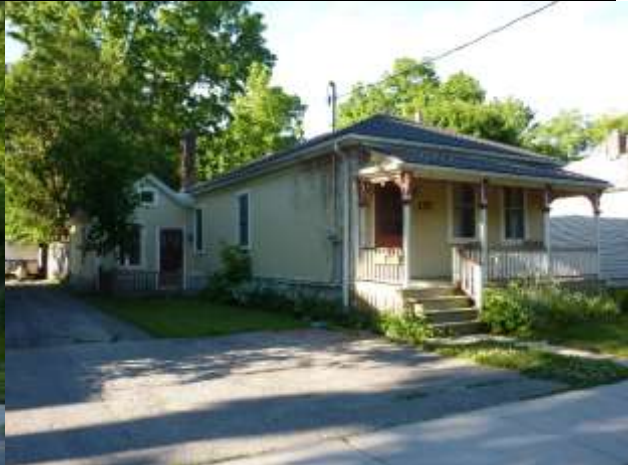
Image 2: Building at 169 Bruce Street (2016-06-14).
