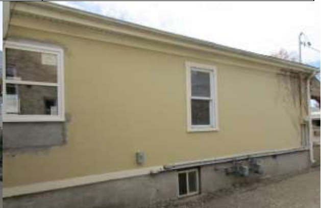
Image 4: Detail of altered window on the east façade (2016-11-10).
