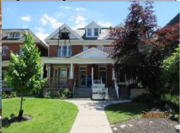
Image 5: Building at 299 Central Avenue.
