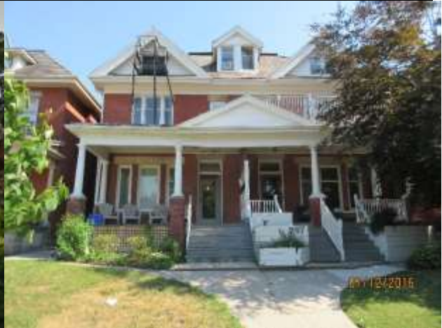
Image 2: Building at 299 Central Avenue.
