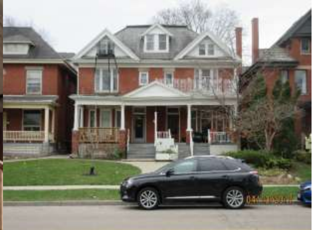
Image 4: Building at 299 Central Avenue.
