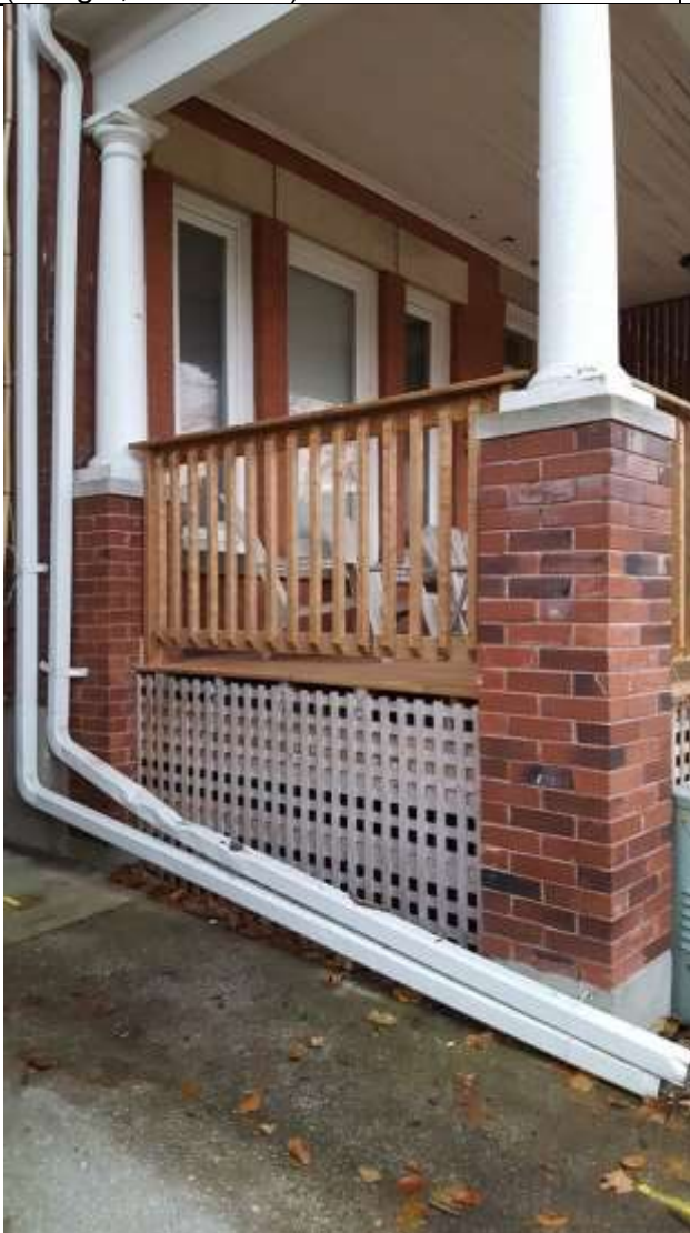
Image 3: New railing at 299 Central Avenue (November 28, 2016).
