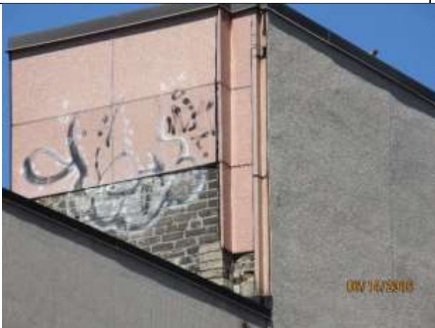
Image 4: Parging of Exterior, 2016
