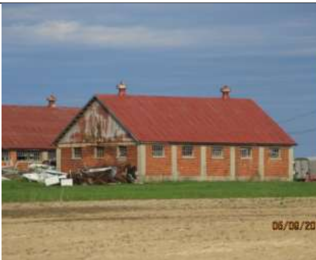
Image 5: The west façade of Barn 3.
