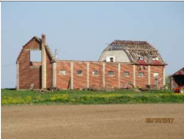
Image 3: Detail of the west façade of Barn 1.
