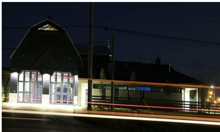
City of Oshawa Fire Station 6
