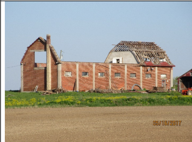
Image 3: Detail of the west façade of Barn 1.
