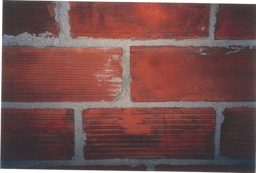
Figure 17: Deterioration on West Side of Northeast Building, 660 Sunningdale Road East
