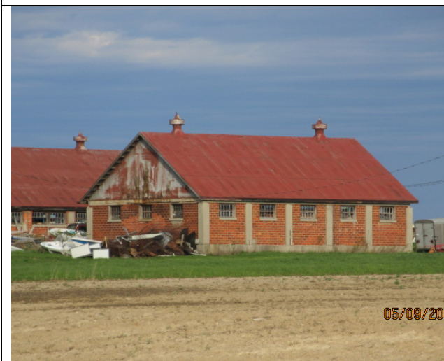
Image 5: The west façade of Barn 3.
