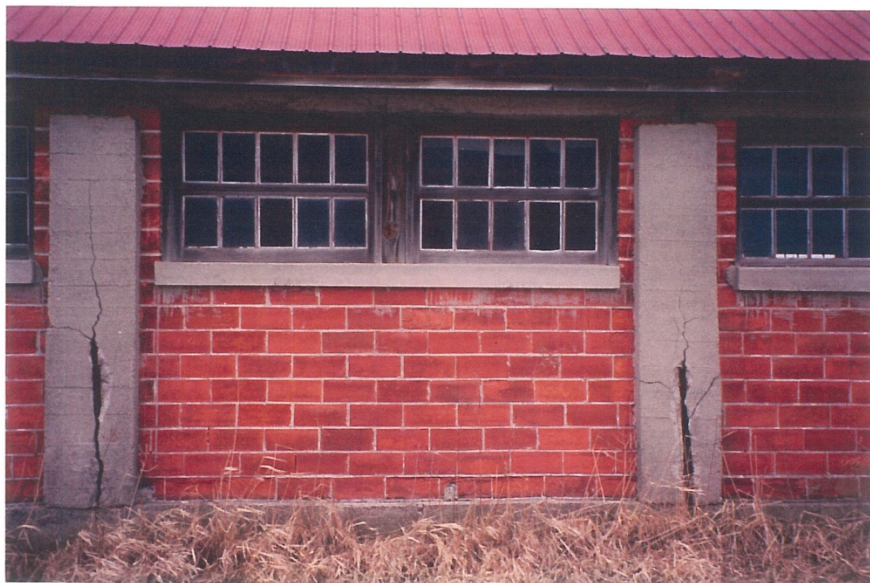
Figure 17: Deterioration on West Side of Northeast Building, 660 Sunningdale Road East
