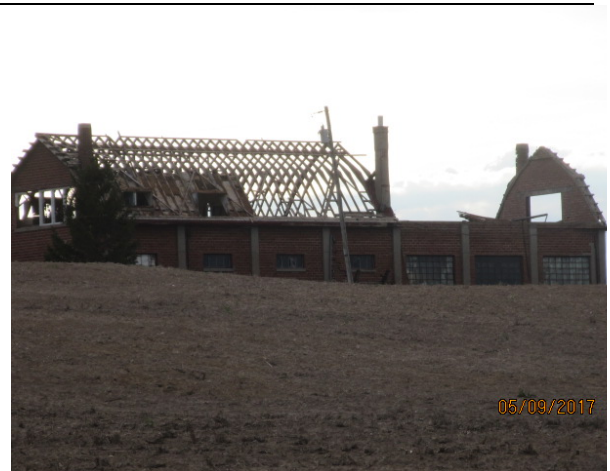
Image 2: Detail the east façade of Barn 1.
