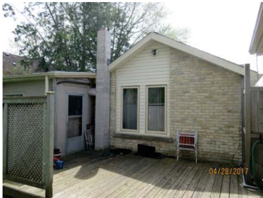
Detail of east (rear) facades
