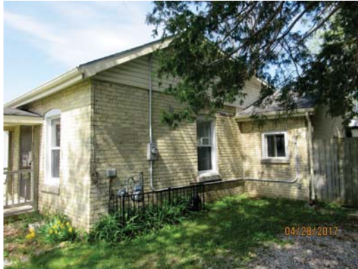
View of south façade showing additions
