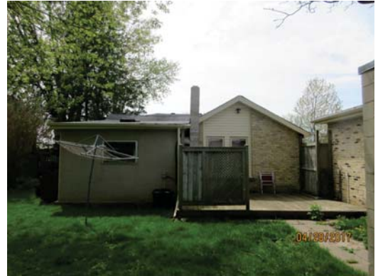
View of east (rear) facades, showing alterations
