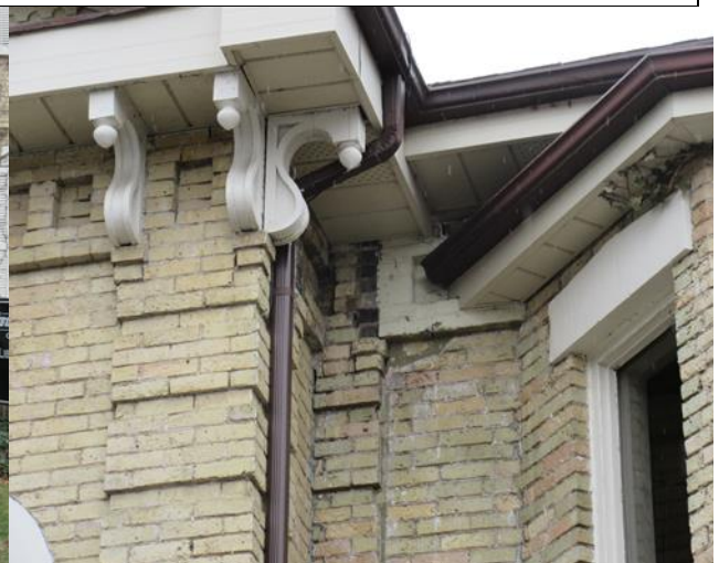
Image 6: North façade detail of soffit, 95 Dufferin Avenue (April 2015)
