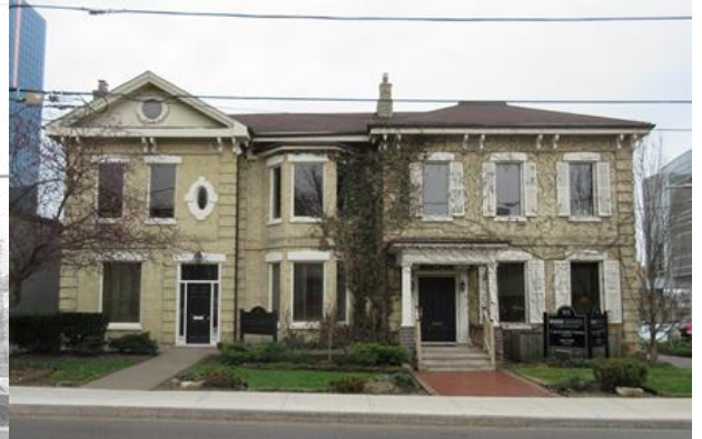
Image 4: North façade of 93-95 Dufferin Avenue showing "double house" composition (April 2015)
