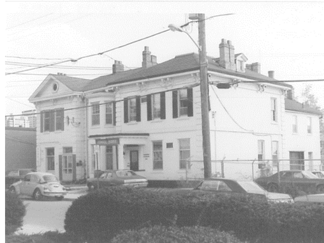
Image 3: North-west facades of 93-95 Dufferin Avenue (date unknown)
