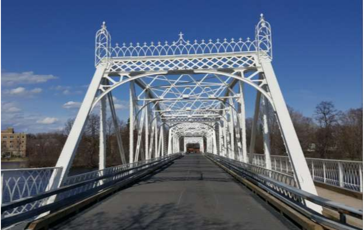
Figure 2 –Minto East Bridge, City of Ottawa –2016
