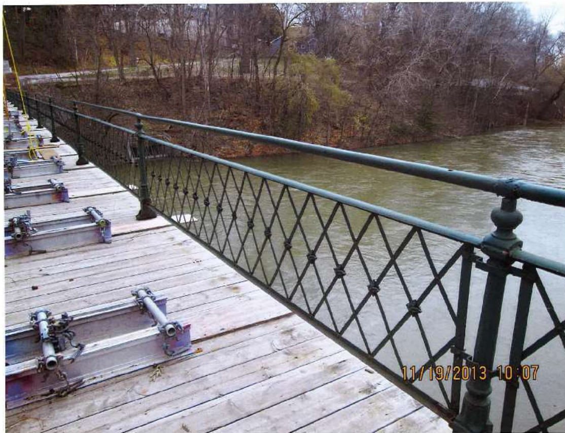
Figure 1 – Blackfriars Bridge – Existing Pedestrian Railing
