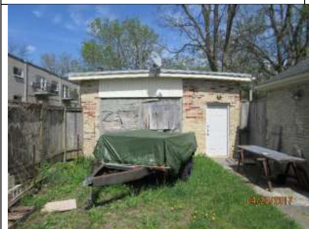
Image 5: Detached garage located at 220 Greenwood Avenue.
