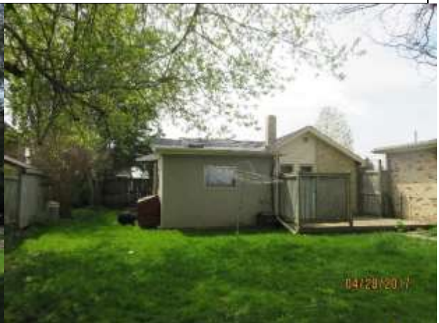
Image 4: Rear (east) façade of the building located at 220 Greenwood Avenue, with garage at right.
