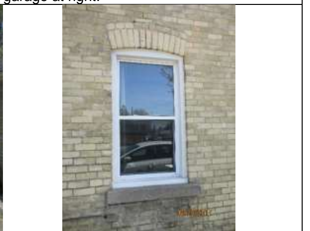
Image 6: Detail of window on the north façade of the building at 220 Greenwood Avenue.
