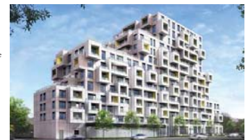
SQ Condominium Building in Alexandra Park Rendering of a new residential building designed by Teeple Architects. The exterior of Alexandra Park Block 11 is only 3 percent glazing, significantly reducing the bird collision hazard posed by this building. Rendering: Teeple Architects
