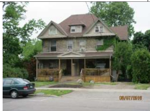
Image 5: Alterations to the verandah at 362 & 364 Princess Avenue.
