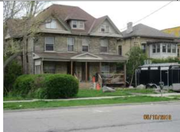
Image 3: Alterations to the verandah at 362 & 364 Princess Avenue underway.
