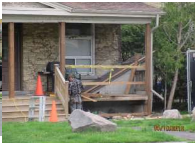
Image 4: Detail of the work underway at 362 & 364 Princess Avenue.
