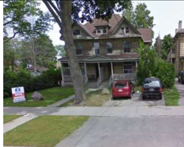
Image 1: Building at 362 & 364 Princess Avenue (Google, July 2009).
