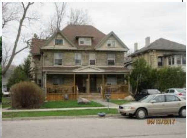
Image 6: Recent photograph of the building at 362 & 364 Princess Avenue.
