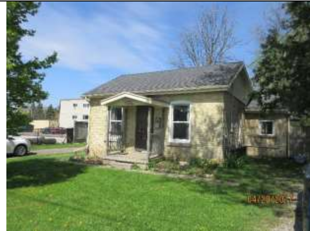
Image 1: Main (west) façade of the building located at 220 Greenwood Avenue.
