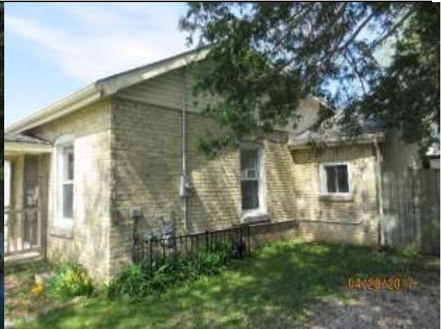
Image 2: South façade of the building at 220 Greenwood Avenue.
