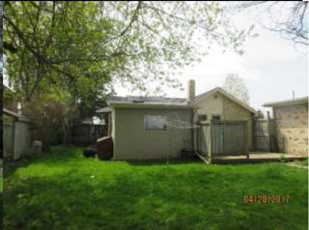
Image 4: Rear (east) façade of the building located at 220 Greenwood Avenue, with garage at right.
