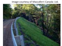
Example of a 1:1 Reinforced Fill Slope
