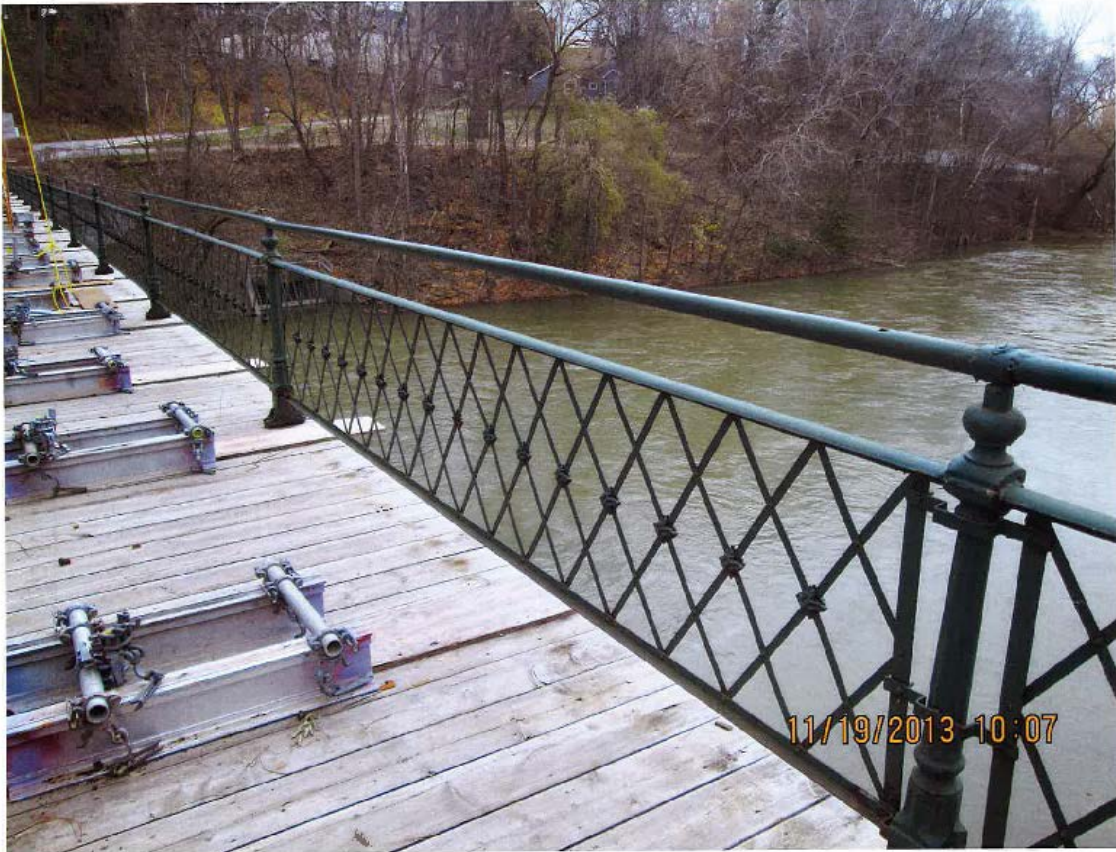
Figure 1 – Blackfriars Bridge – Existing Pedestrian Railing
