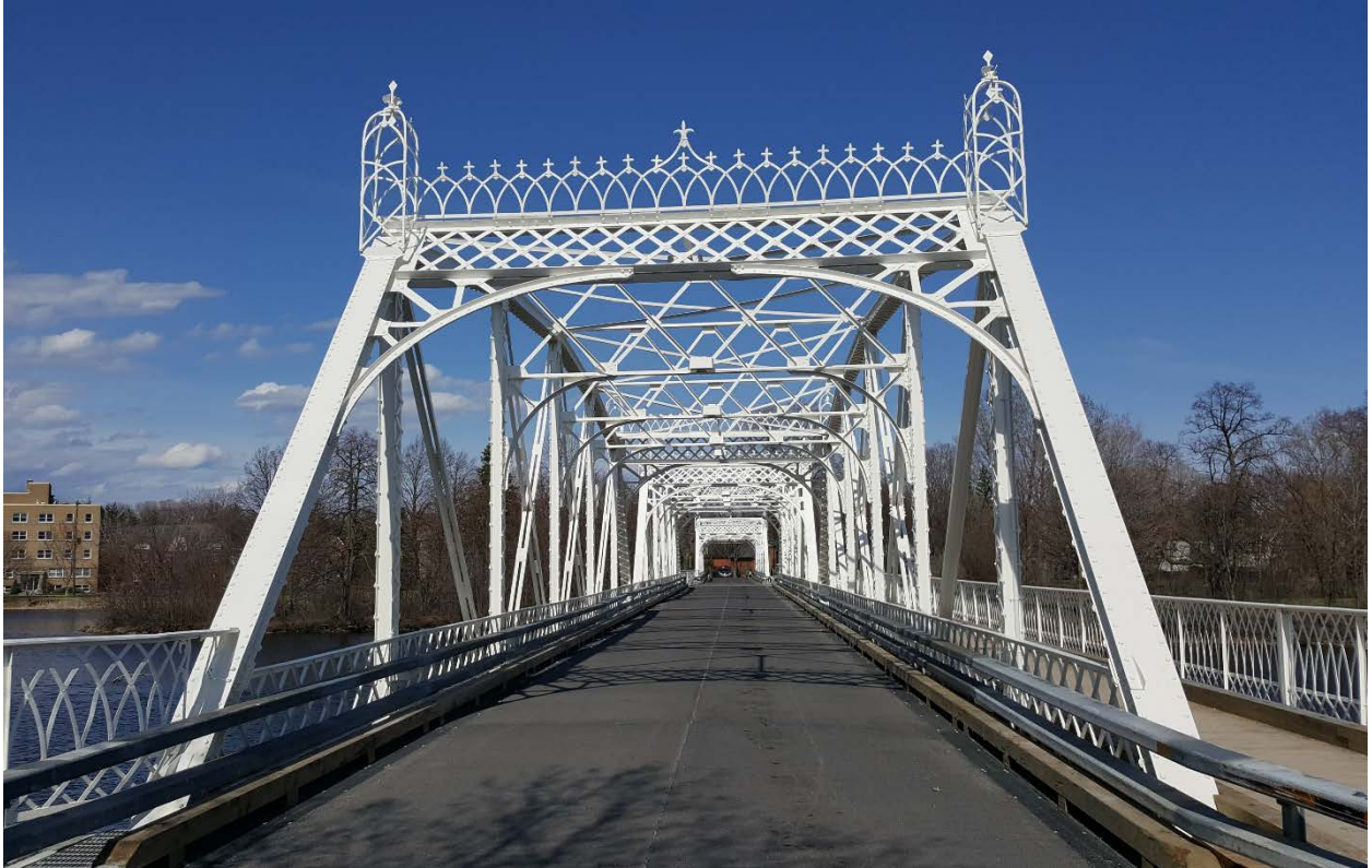
Figure 2 –Minto East Bridge, City of Ottawa –2016
