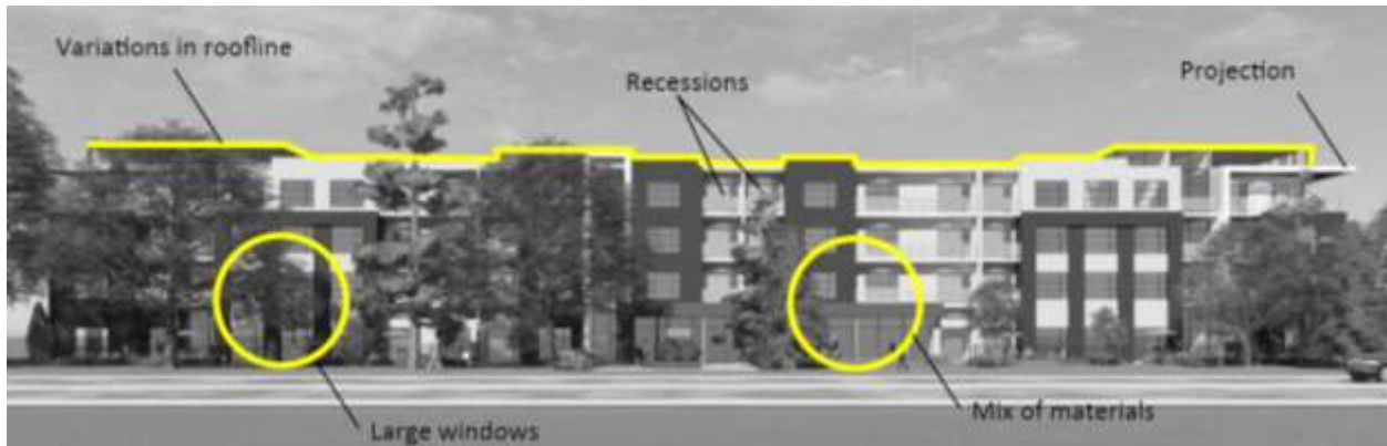
Figure 7: South Building Façade
