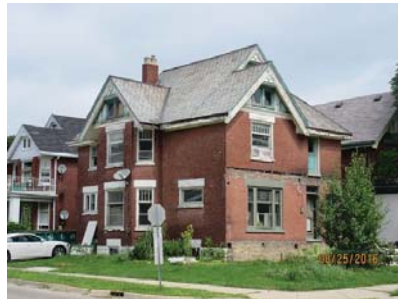
porch removed prior to August 25 th 2016
