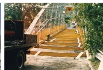
Blackfriars Bridge (during 1980s rehabilitation)
