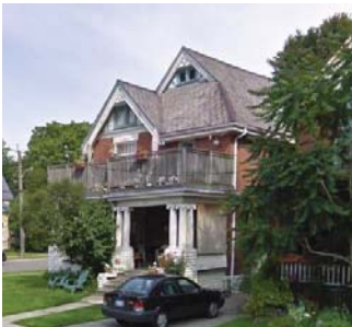
existing porch with original porch detailing (cast concrete columns, concrete piers, solid wood porch rails)
