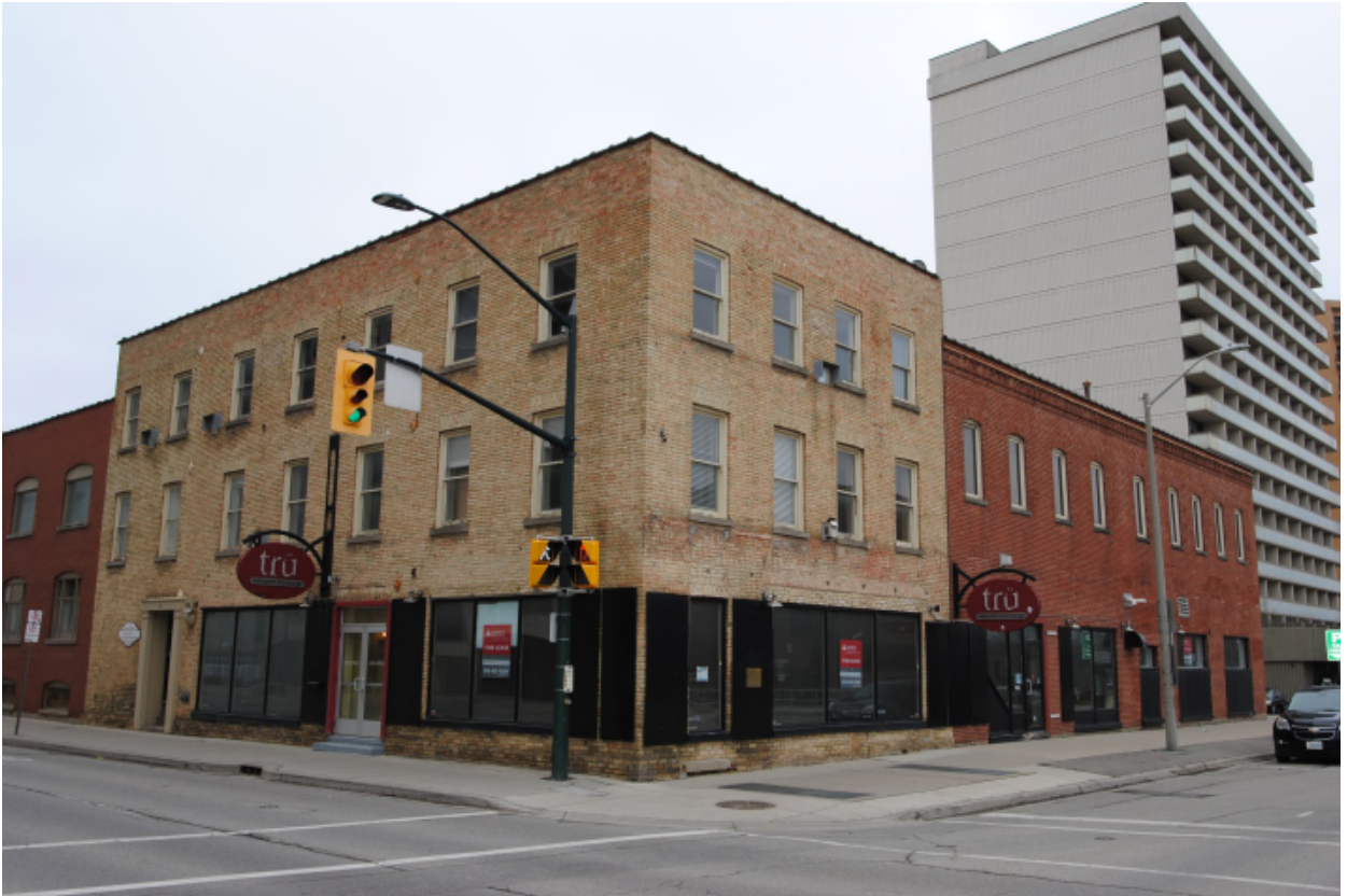
359 Ridout Street formally 363 Ridout St. Photo Credit: Nicholson Sheffield Architects Inc.
