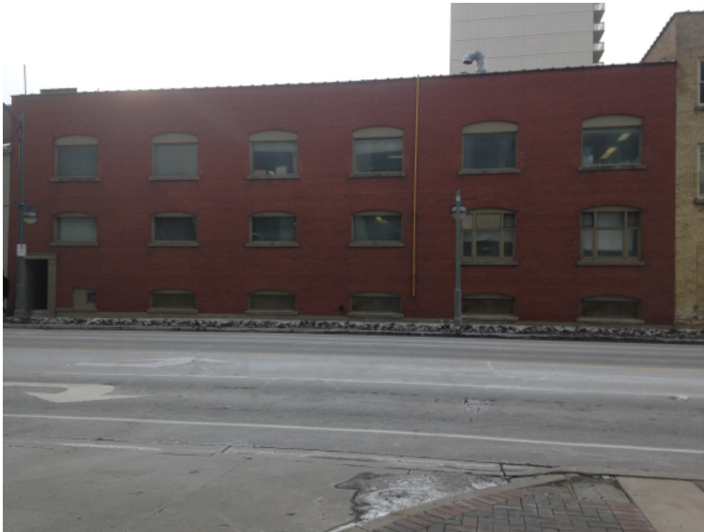
355 Ridout Street East Elevation, Photo Credit Nicholson Sheffield Architects Inc.
