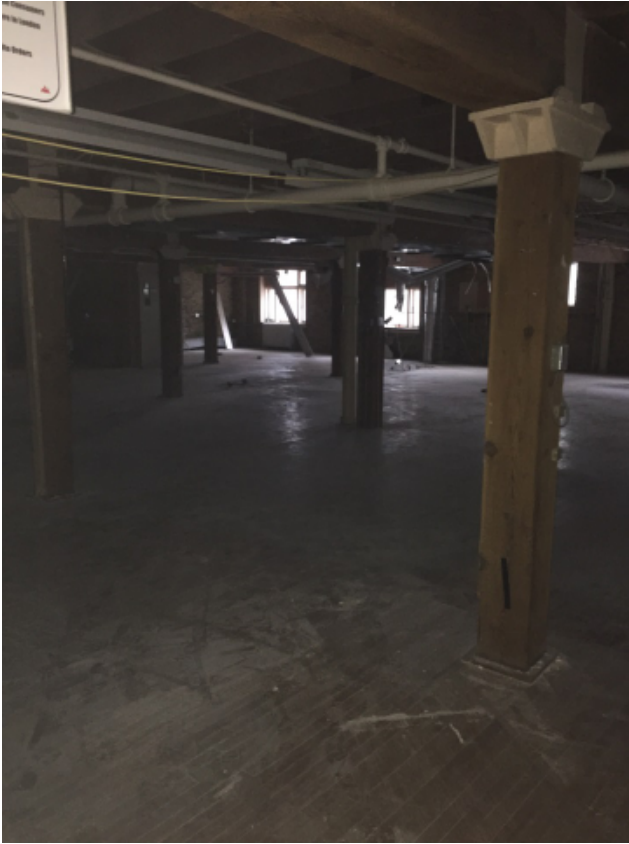
355 Ridout Street First Floor, Photo Credit Nicholson Sheffield Architects Inc.
