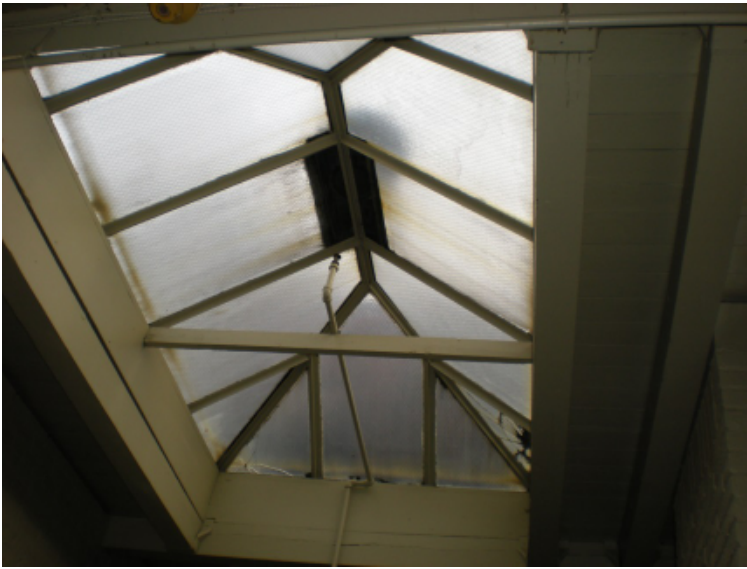
341 Ridout Sky light Detail, Photo Credit Nicholson Sheffield Architects Inc.
