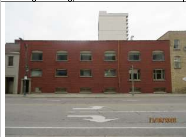
Image 5: 355 Ridout Street North (former Jenkins Warehouse).
