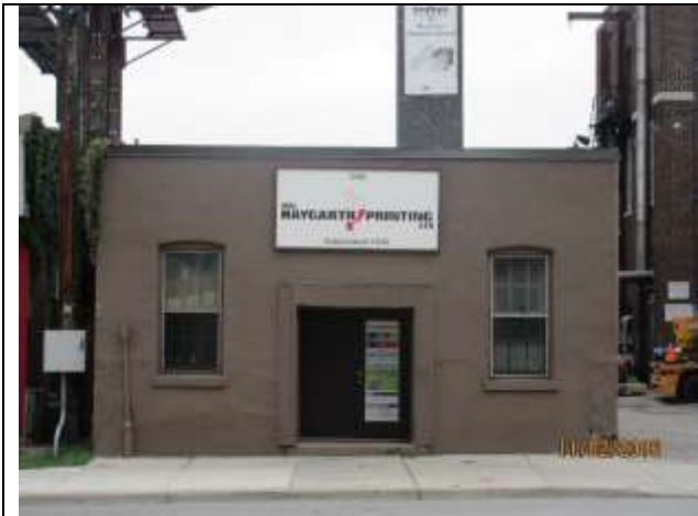
Image 1: 345 Ridout Street North (former Haygarth Printing Ltd.)
