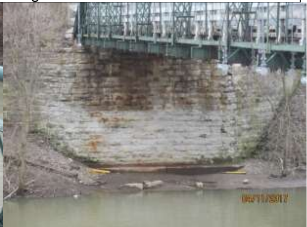
Image 12: Detail of (east) stone abutment of Blackfriars Bridge.
