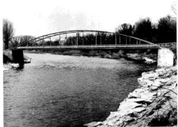
Image 4: View of Blackfriars Bridge, circa 1930 (courtesy London Room).
