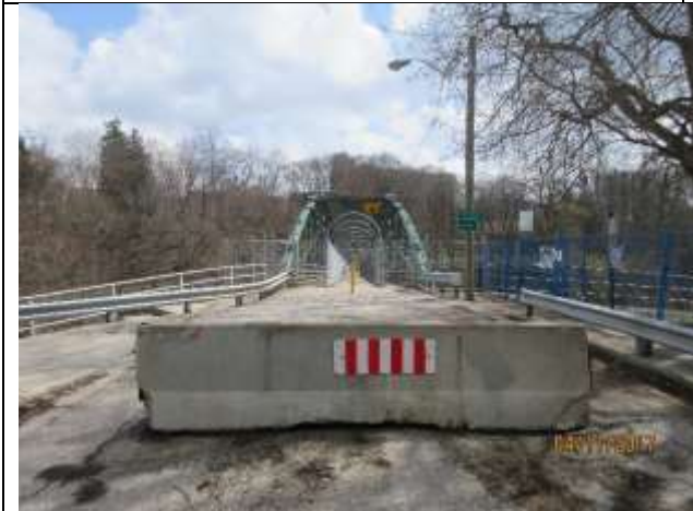
Image 9: West approach to Blackfriars Bridge.
