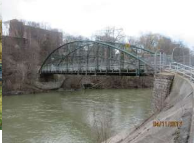
Image 8: View looking southeast of Blackfriars Bridge.
