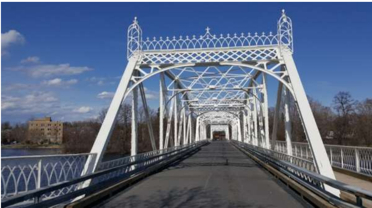
Image 1: Minto East Bridge on April 23, 2017 (courtesy Dillon).
