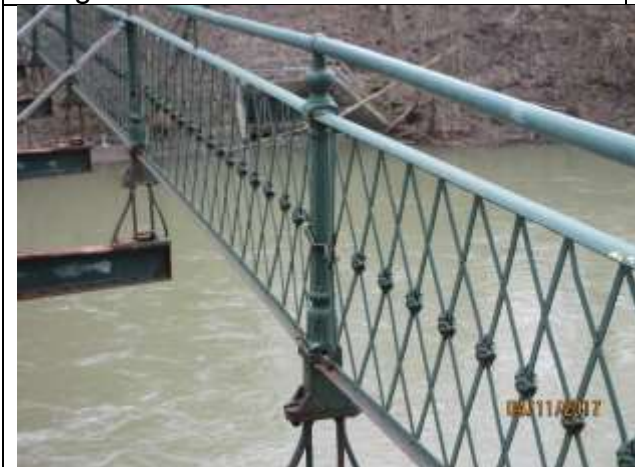
Image 11: Detail of existing pedestrian guard/hand railing.
