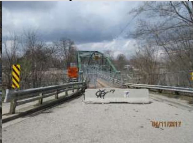
Image 10: East approach to Blackfriars Bridge.
