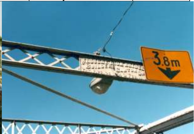
Image 6: Detail of Wrought Iron Bridge Company sign (1983).
