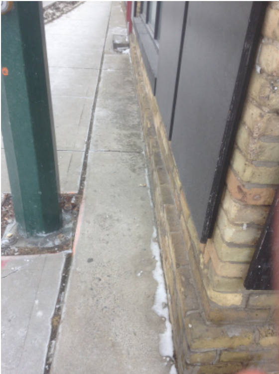
45 King Street, Photo Credit Nicholson Sheffield Architects Inc.
