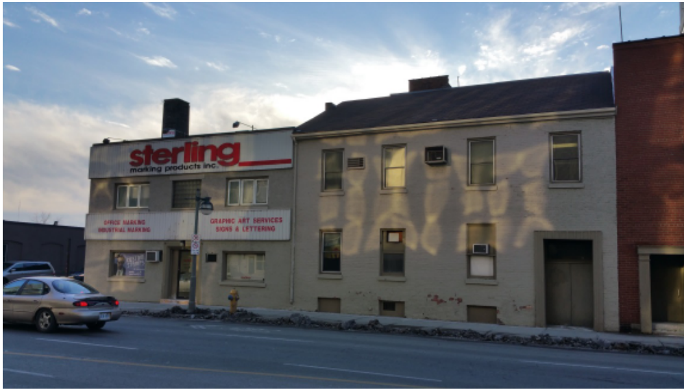
351 Ridout Street c. 1880, Photo Credit Nicholson Sheffield Architects Inc.
