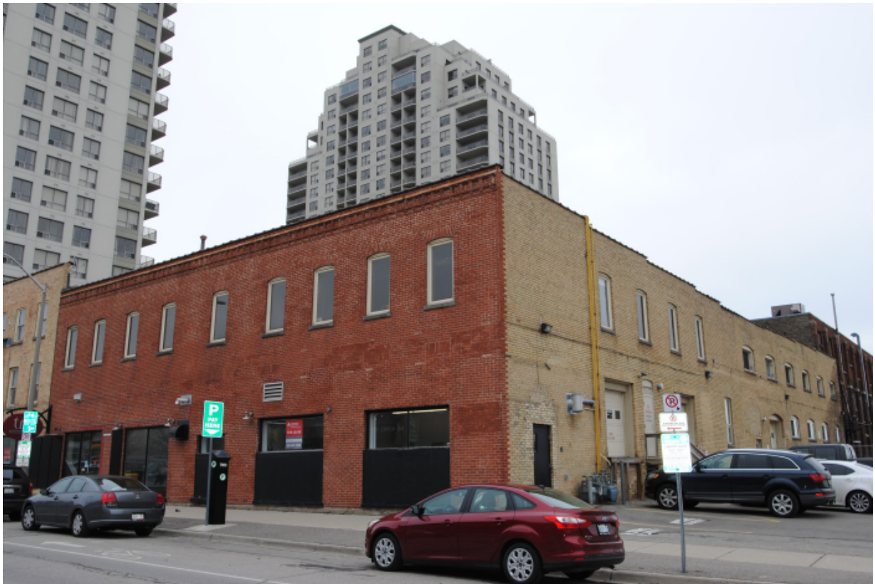
45 King Street. Photo Credit: Nicholson Sheffield Architects Inc.
