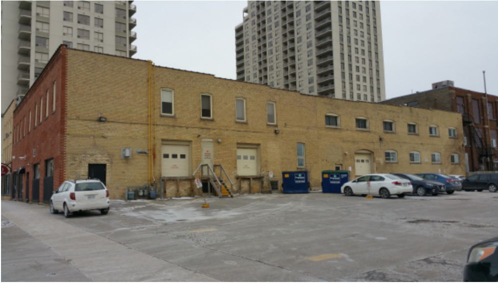
45 King Street, Photo Credit Nicholson Sheffield Architects Inc.
