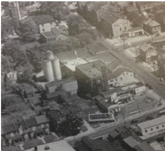
North-east corner of Ridout and York Streets, c 1946, therefore the current form of the site is represented as it is today. (Source: Downtown London Layers of Time.)
