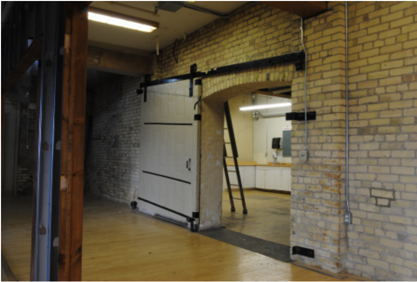
45 King 1922 Addition Second Floor Photo Credit Nicholson Sheffield Architects Inc.
