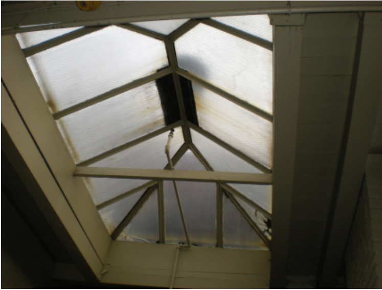
341 Ridout Sky light Detail, Photo Credit Nicholson Sheffield Architects Inc.
