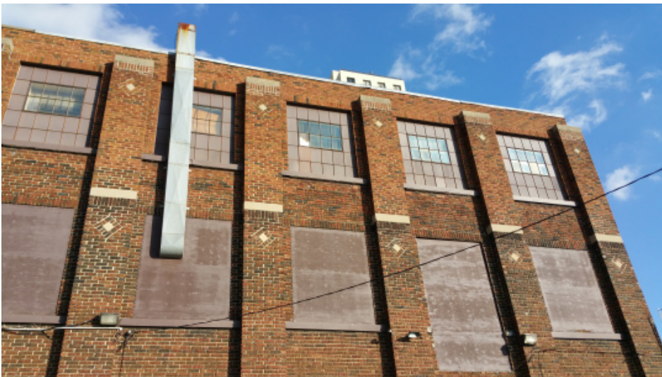
341 Ridout Street West Elevation, Photo Credit Nicholson Sheffield Architects Inc.
