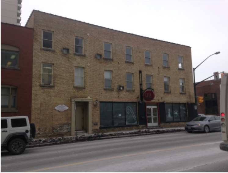
363 Ridout Street, Photo Credit Nicholson Sheffield Architects Inc.
