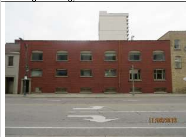
Image 5: 355 Ridout Street North (former Jenkins Warehouse).
