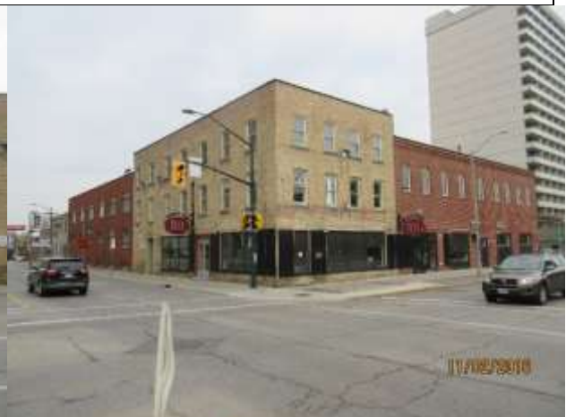
Image 6: 359 Ridout Street North (former McFarlane Hotel/Grand Central Hotel).
