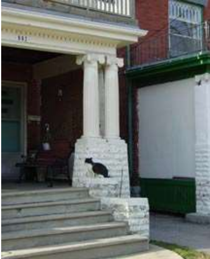
APPENDIX F — Example of fabricated finger jointed wood column with Tuscan capital
