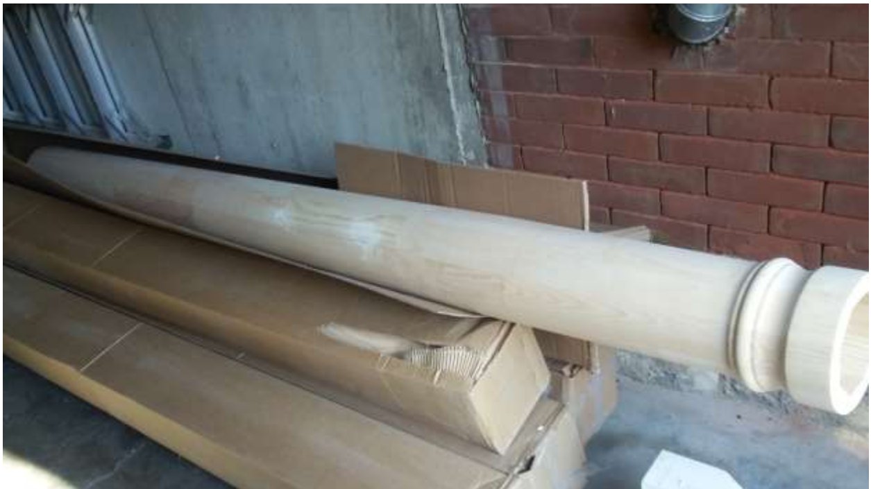
APPENDIX F — Example of fabricated finger jointed wood column with Tuscan capital
