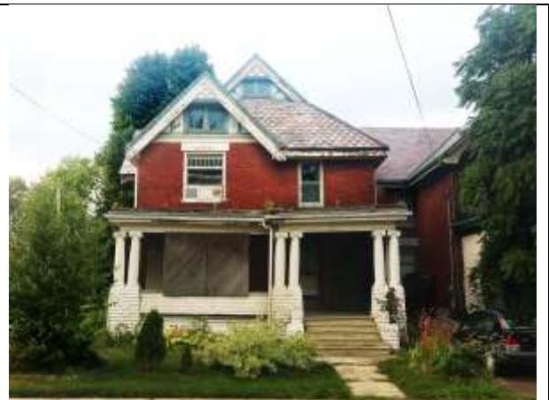
Image 2: Front façade showing porch prior to demolition (photo by owner)
