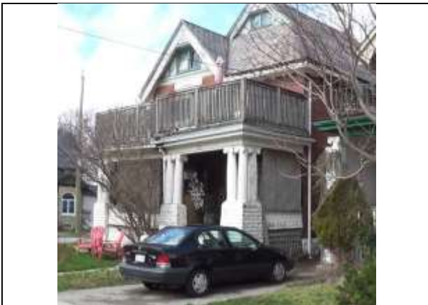
Image 1: Front façade showing porch prior to demolition (photo by owner)
