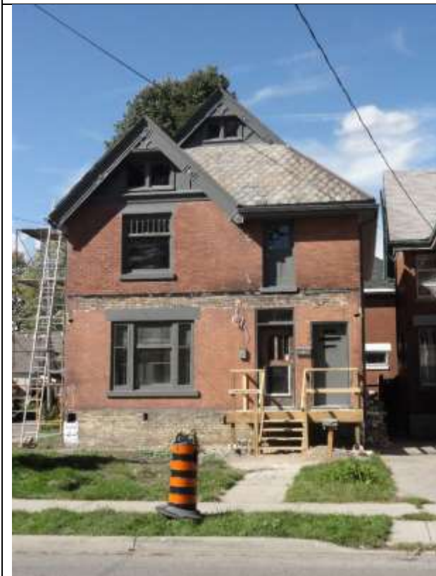
Image 3: Front façade showing removal of existing porch
