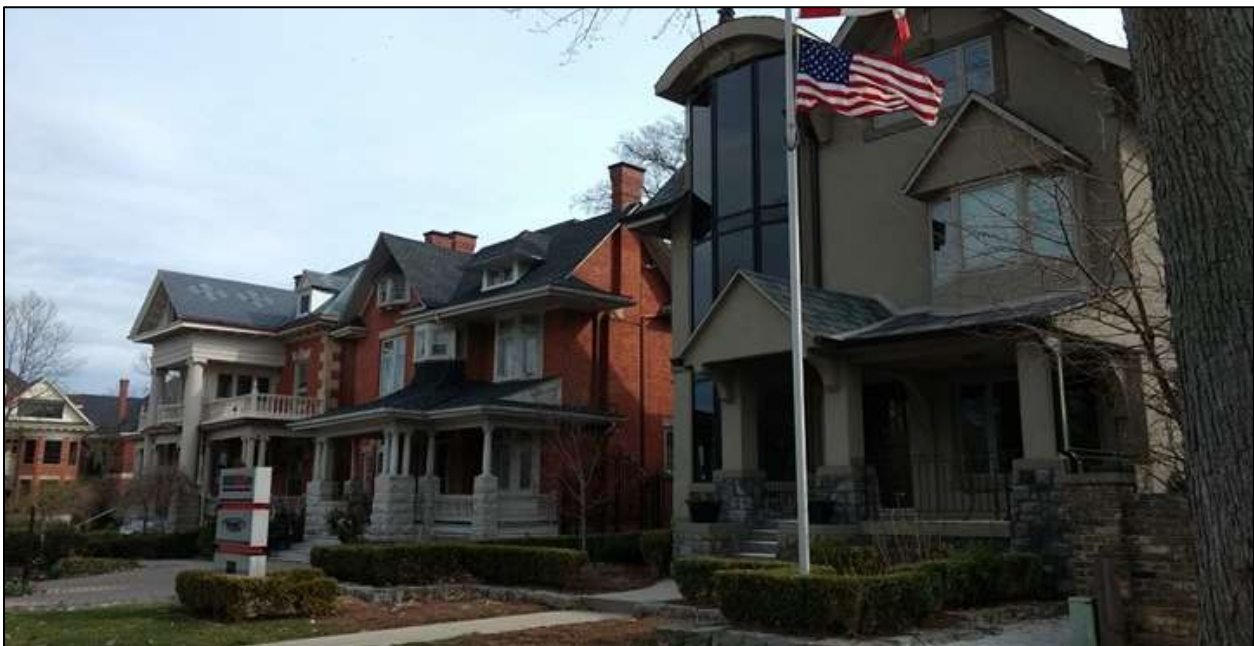
Figure 9 – Adjacent built form on Wellington Street
