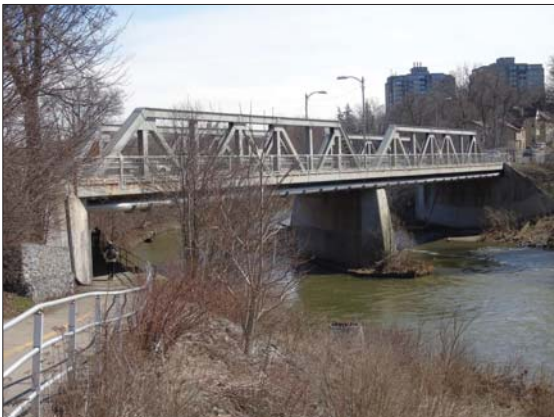
Riveted, modified Warren truss structure with seven panels
