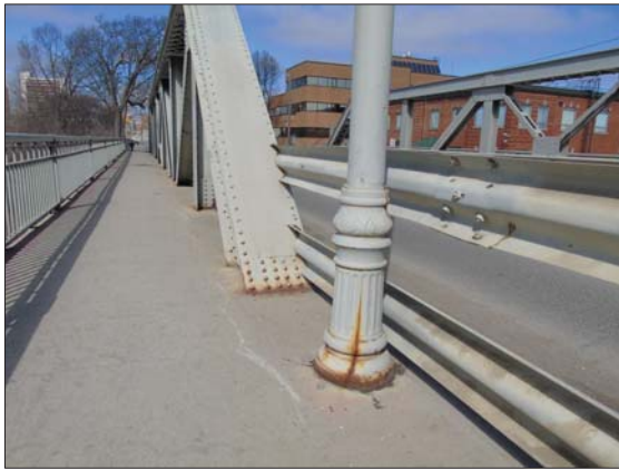
Decorative lamp posts in centre of the bridge spans
