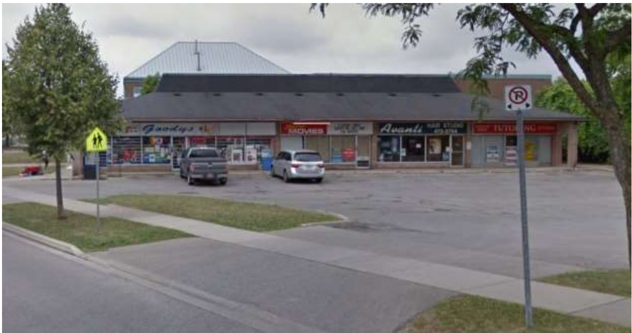
Figure 2 –Easterly Façade of Existing Commercial Building.
