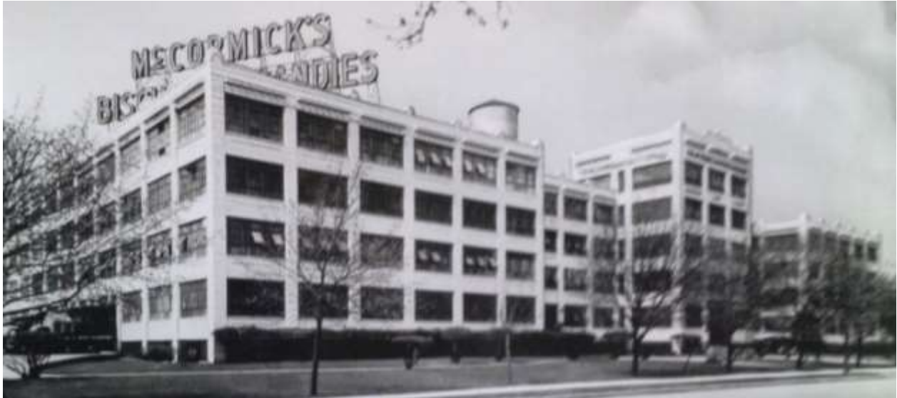
Original McCormick's Factory Building showing Dundas Street façade of five story centre block and location of decorative parapet terra cotta. (Source: June 23, 2015 Heritage Impact Assessment)
