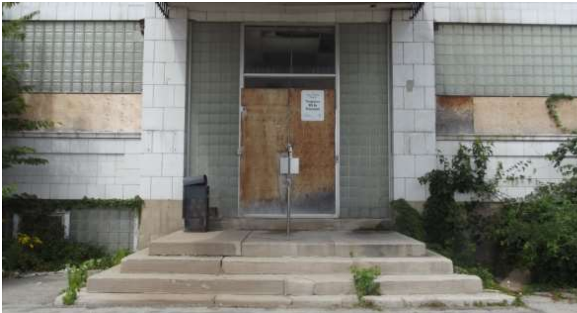
Existing condition of central main entrance to original McCormick Factory building (2015)
