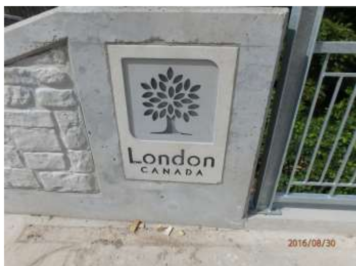
Figure 9 – Stoney Creek Bridge
