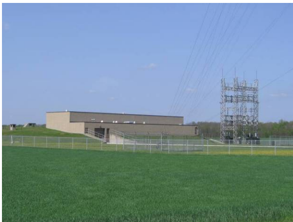
Figure 1: McGillivray Booster Pumping Station
