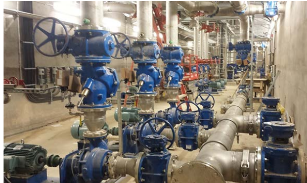
Figure 4e: Pipe Gallery
