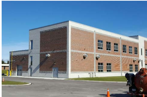
Figure 4c: Residuals Management Facility – northeast elevation.
