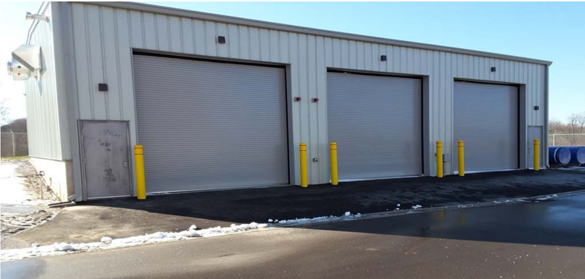
Figure 5: Exterior of the new storage building.
