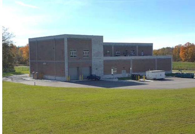
Figure 4b: Residuals Management Facility – southwest elevation.
