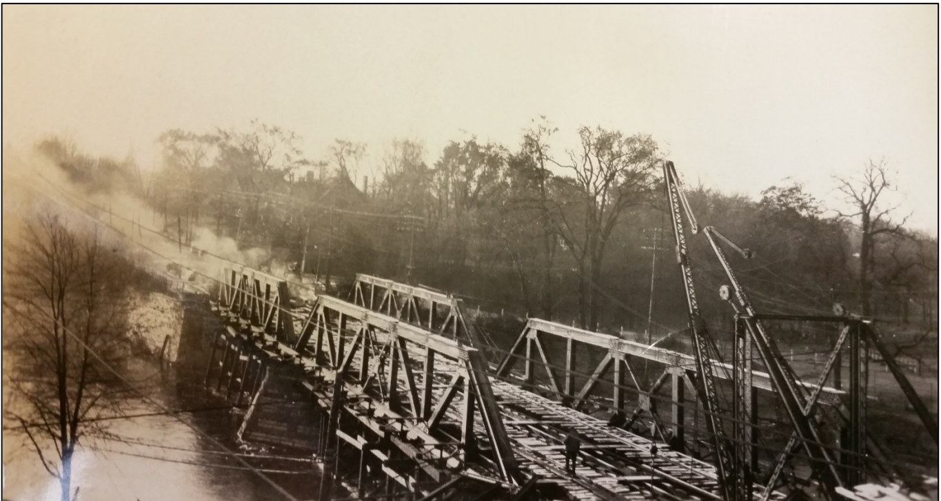
Photograph 7: Victoria Bridge under construction in 1925 (Victoria Bridge Clippings File, London Room)
