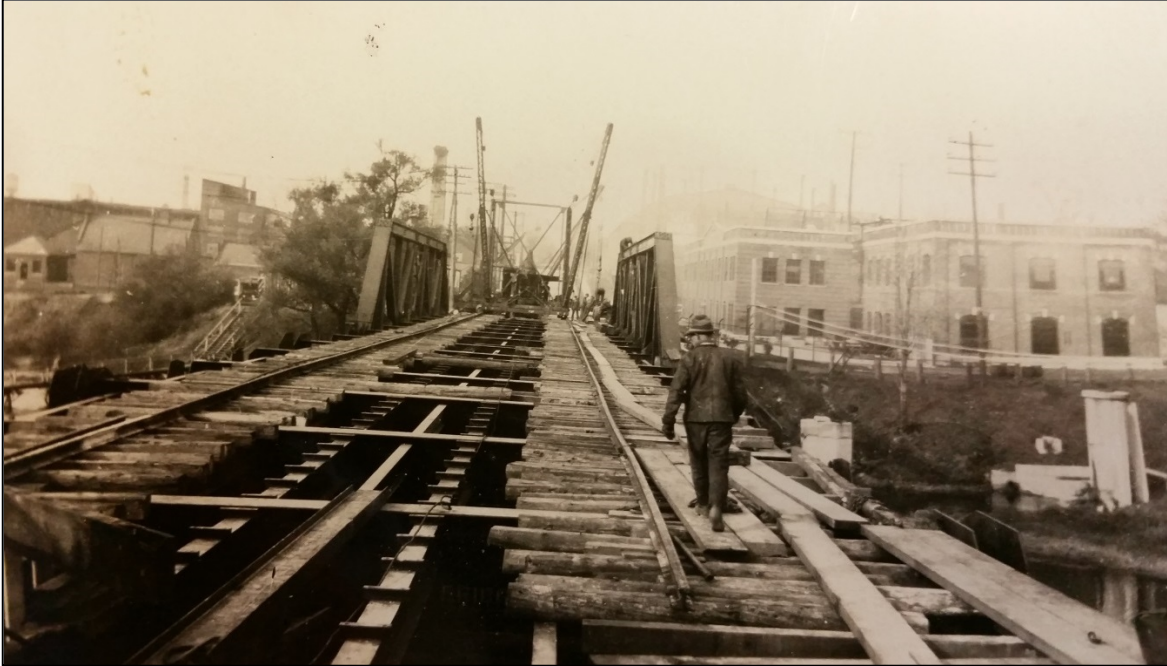
Photograph 4: Victoria Bridge under construction in 1925 (Victoria Bridge Clippings File, London Room)
