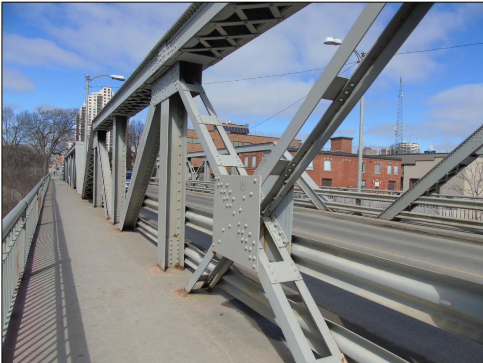
Photograph 11: Riveted truss panels, identified as a Heritage Attribute
