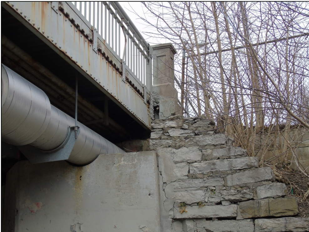
Photograph 13: View of remnant concrete and stone endpost at the north approach to the bridge, identified as a Heritage Attribute
