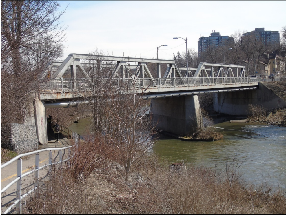
Photograph 10: West side of Victoria Bridge showing Warren truss, identified as a Heritage Attribute
