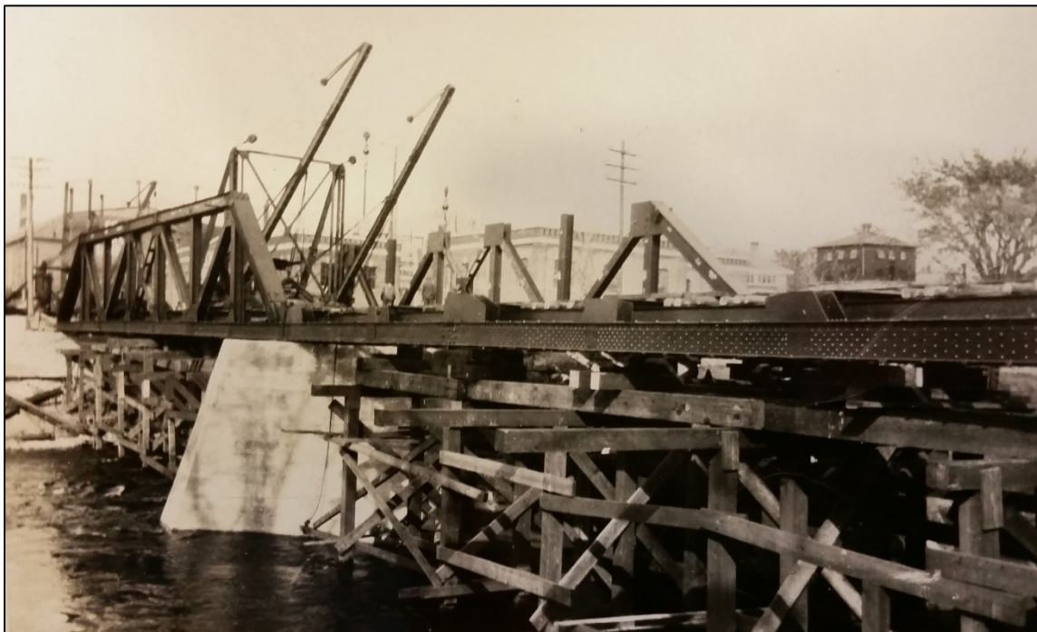
Photograph 3: Victoria Bridge under construction in 1925 (Victoria Bridge Clippings File, London Room)
