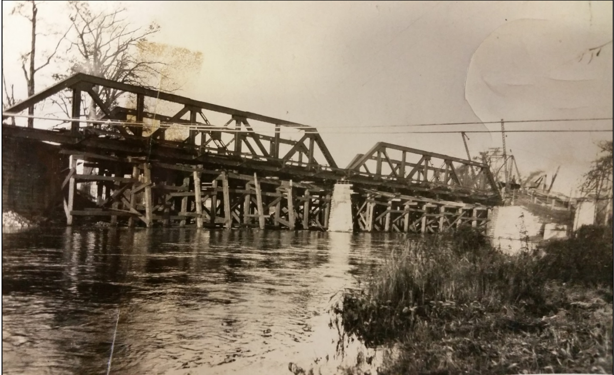
Photograph 6: Victoria Bridge under construction in 1925, showing temporary trestle structure under the bridge during construction (Victoria Bridge Clippings File, London Room)
