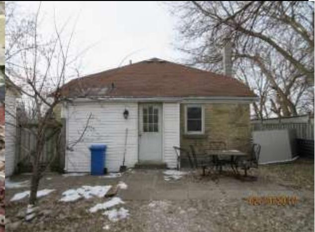
Image 4: Rear (east) façade of the building located at 34 Muir Street.
