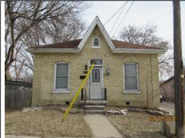
Image 1: Main (west) façade of the building located at 34 Muir Street.
