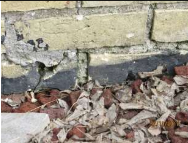
Image 3: Evidence of previous paint on the brick of the building at 34 Muir Street.
