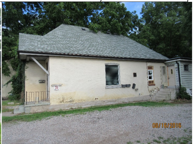
Image 2: West façade of the building located at 30 Oxford Street West.
