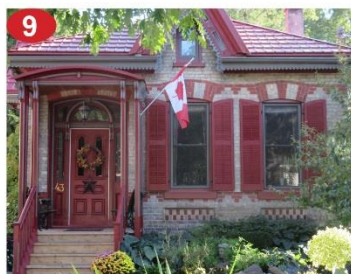
Original brick voids
