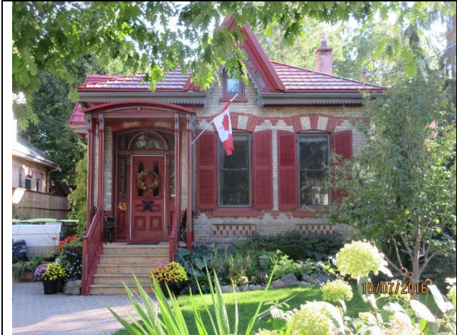
Image 1: Main (north) façade of the building located at 43 Bruce Street.
