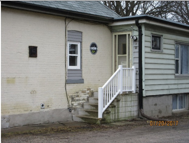
Image 5: Detail of window replacement on west façade of the building located at 30 Oxford Street West.
