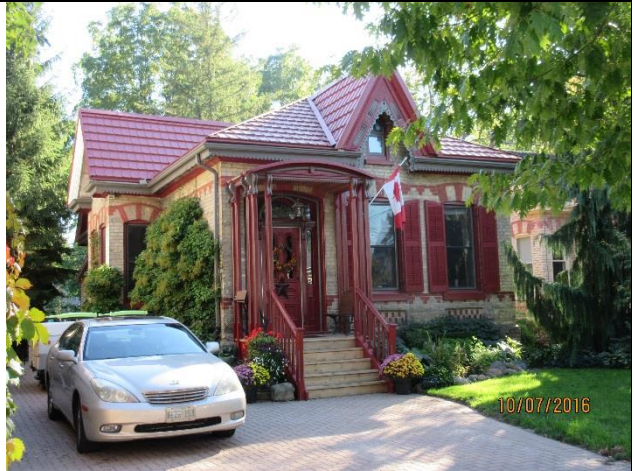
Image 2: East and north facades of the building located at 43 Bruce Street.
