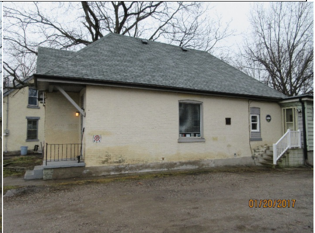
Image 4: West façade of the building located at 30 Oxford Street West.
