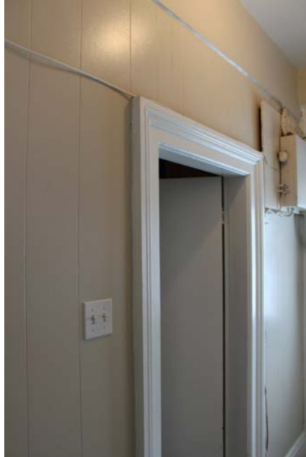
13. Entry wall with painted plywood paneling.
