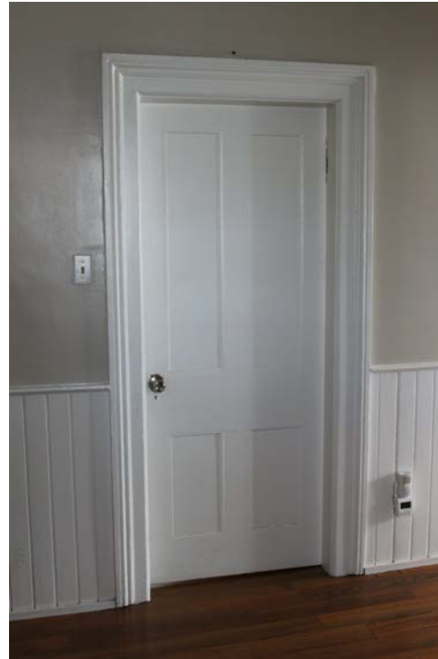
11. Door, door casing and v-match wainscoting. All are thought to be original.
