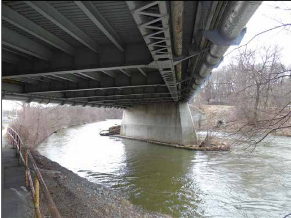
Photograph 34: View of riveted lattice connecting the steel on the bottom chord and the conduits and pipes extending along the west side of the bridge
