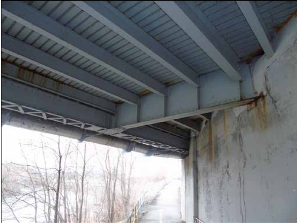
Photograph 32: Underside of deck at north abutments showing deck tray, stringers, and cross beams
