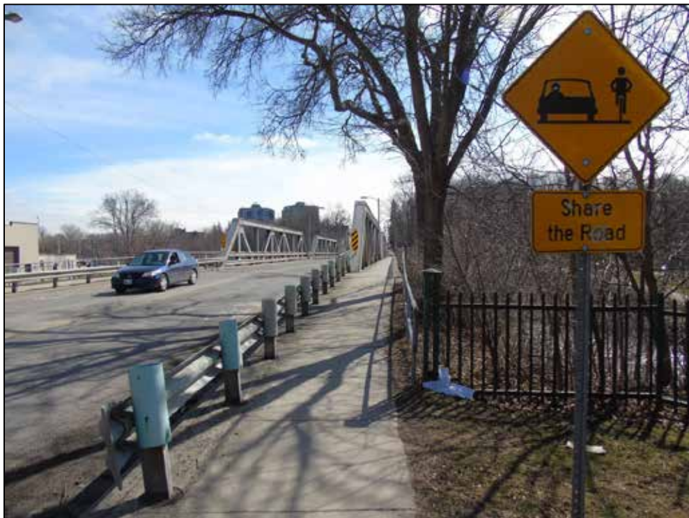
Photograph 19: North approach showing sidewalks and slight grade change at truss
