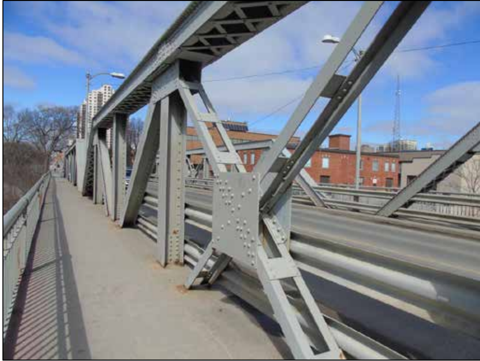
Photograph 28: Viewing showing centre panel with diagonals forming an “X” as part of the modified Warren truss
