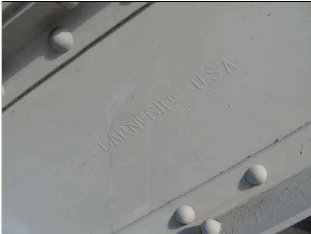
Photograph 31: "CARNEGIE" stamp found throughout the steel used on the truss
