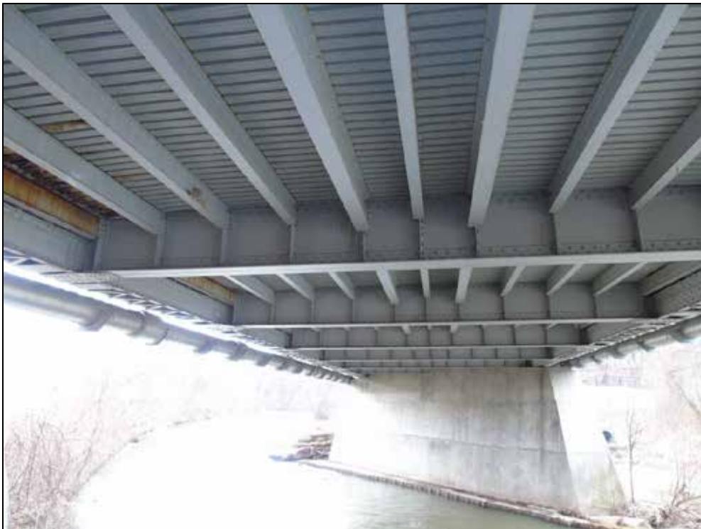
Photograph 33: Viewing looking south showing stringers and cross beams
