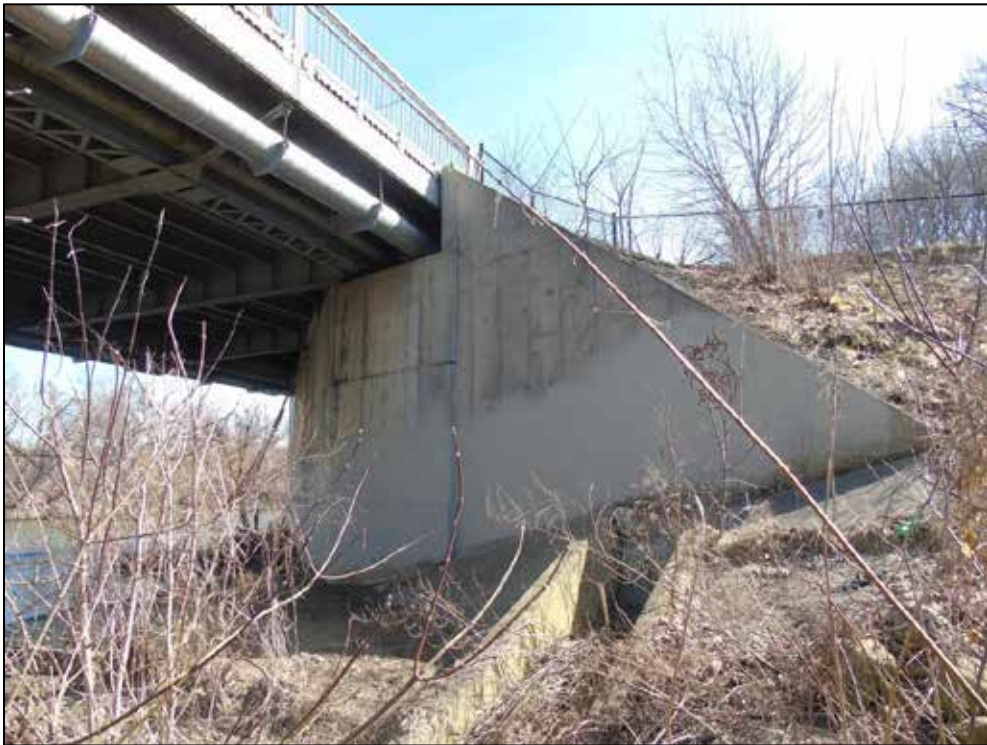
Photograph 25: South abutment, west side, showing embankment and retaining wall
