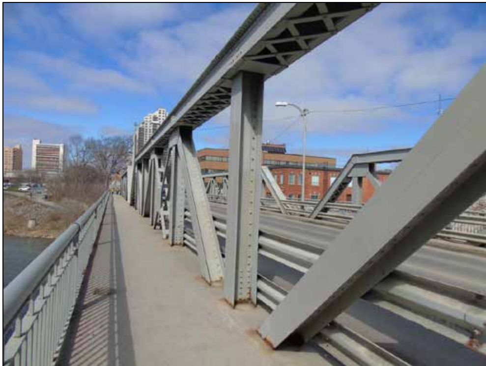
Photograph 27: View showing vertical and diagonal members and top chord with riveted lattice
