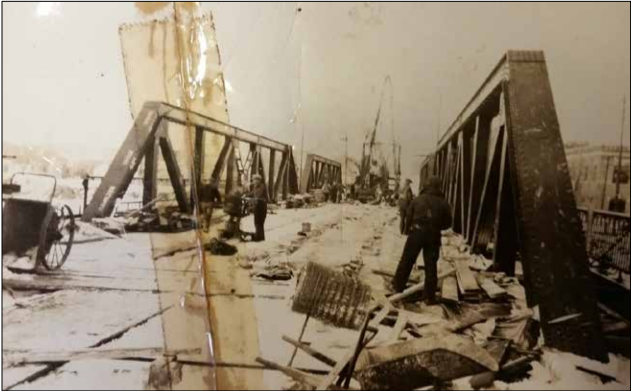
Photograph 9: Victoria Bridge under construction in 1925 showing trusses nearing completion
