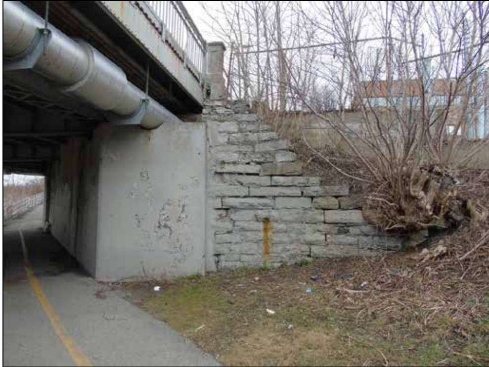
Photograph 22: North embankment, east side, showing remnants of original stone abutment and stone/concrete end post above
