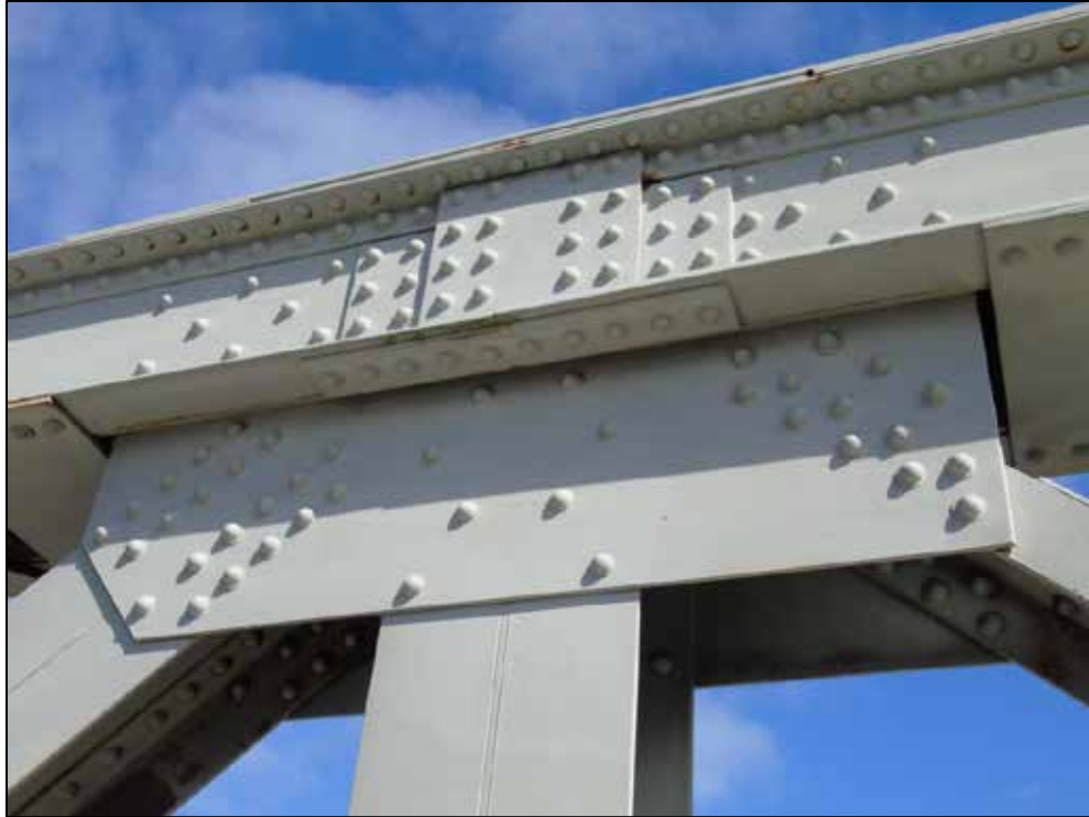
Photograph 30: Connection on top chord showing gusset plates and connection of vertical and diagonal members
