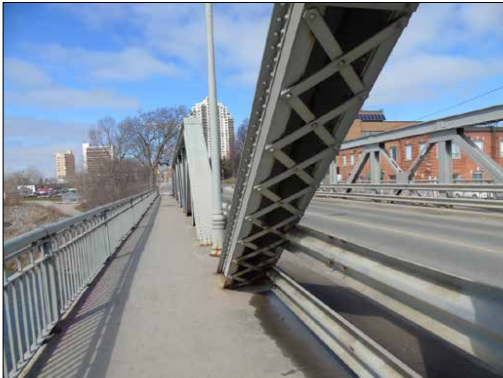
Photograph 29: Viewing showing riveted lattice under the diagonal end posts and decorative lamp posts in between trusses
