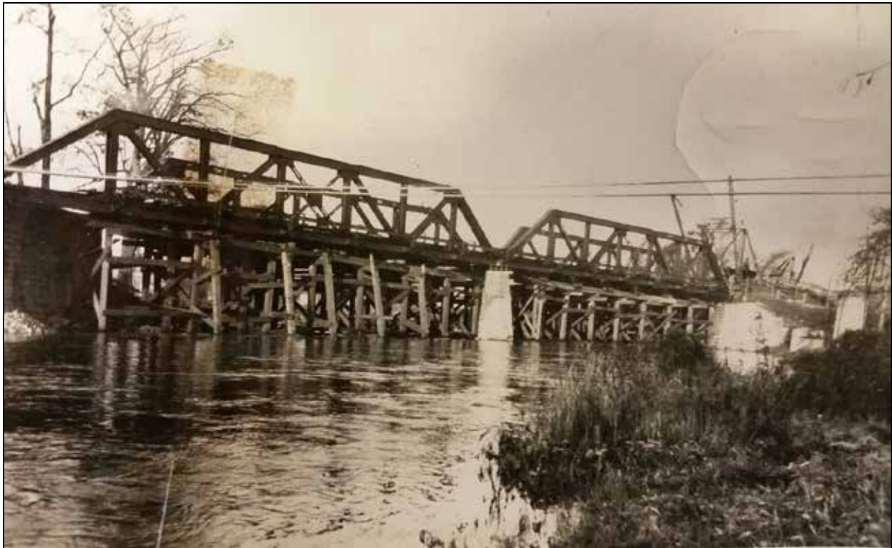
Photograph 10: Victoria Bridge under construction in 1925, showing temporary trestle structure under the bridge during construction
